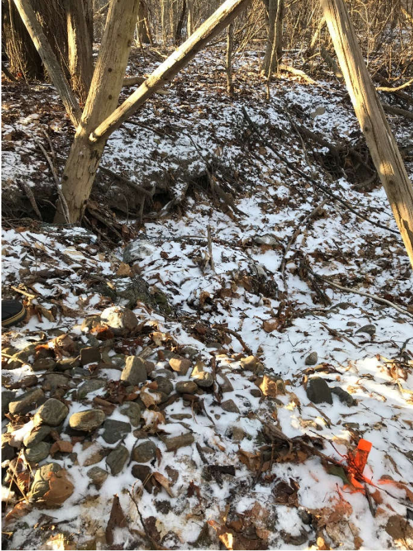
Photo No.1 Gabion Basket Drop Structure
