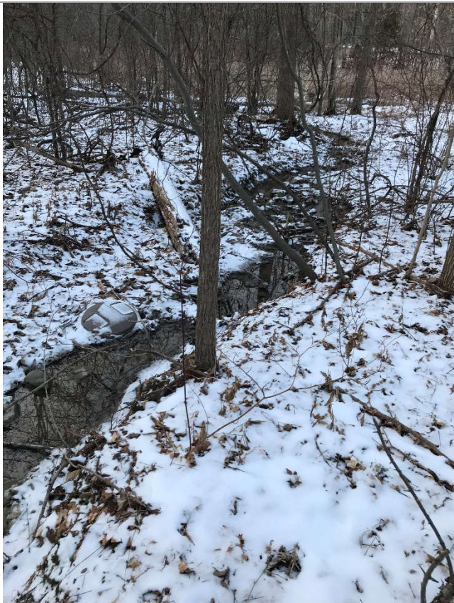
Photo No.3 Channel between gabion basket drop structure and wetland
