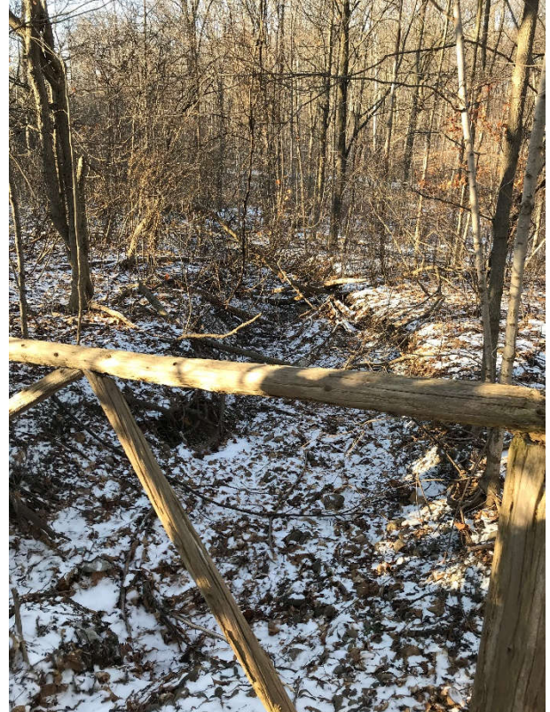
Photo No.2 Channel downstream of gabion basket drop structure
