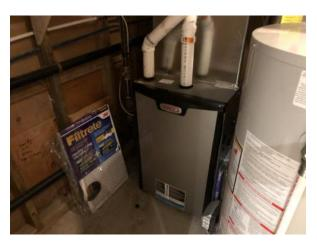
Photo 2: View of the typical natural gas fired furnace observed in all residential properties accessed on Site.
