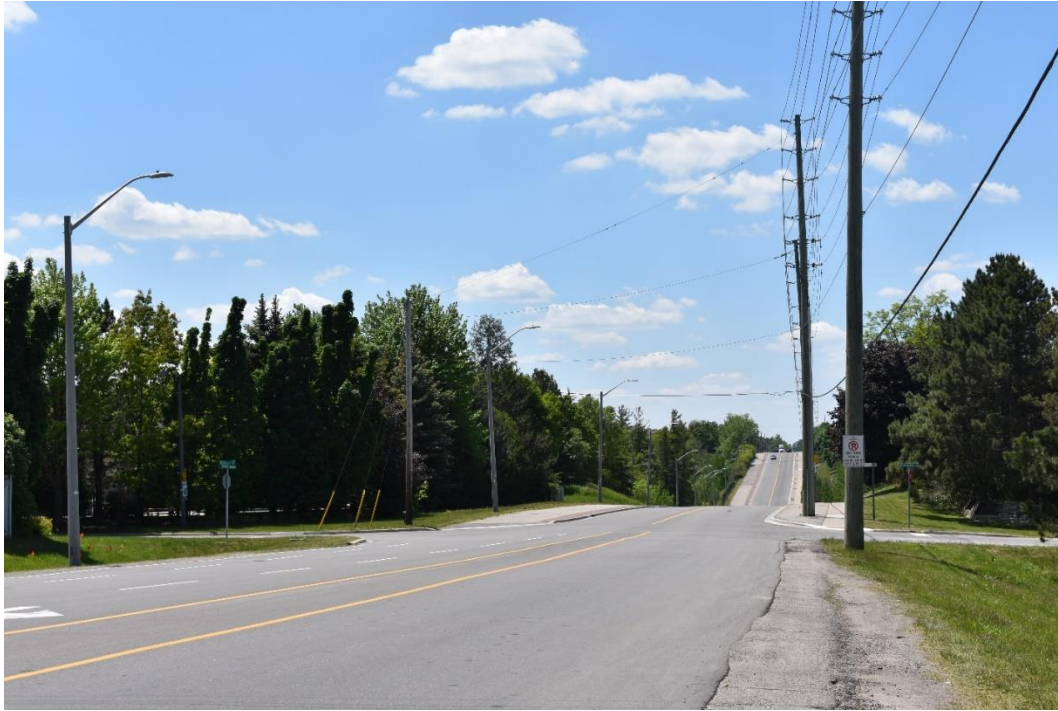
Figure 7 – View from Vandorf Sideroad Looking West. (View of the intersection of Vandorf Sideroad/ Archerhill Court/ Monkman Court; Archerhill Court aligns with Monkman Court)
