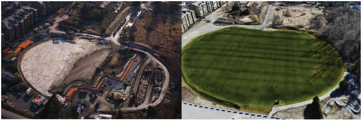
Figure 1: Before and after. Upon completion, this is now one of the largest underground stormwater detention systems in North America.
