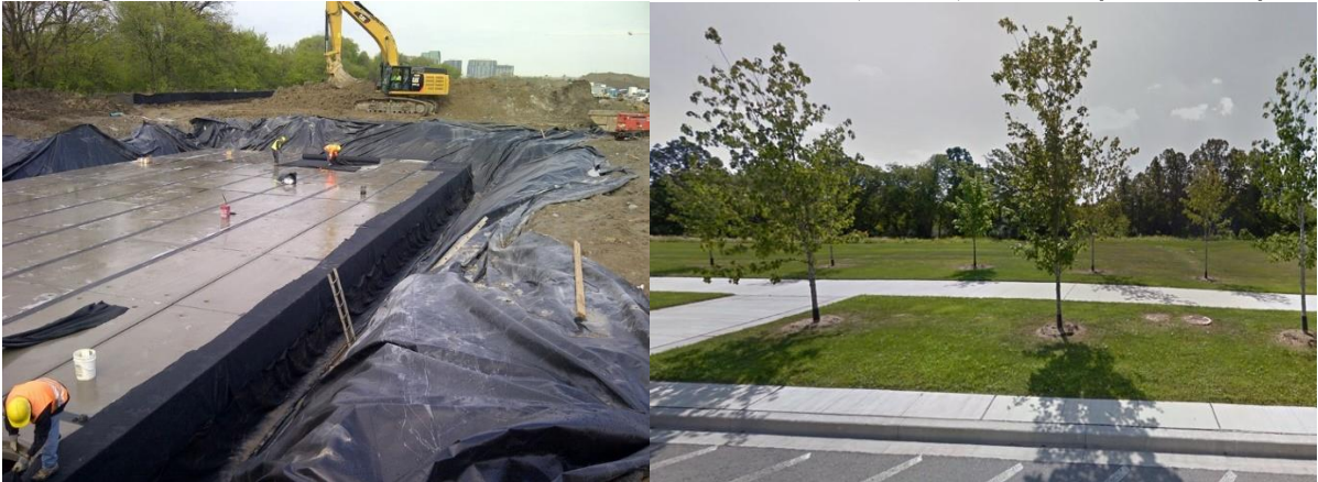
Underground concrete tank construction in Markham (Times) – After park on top
