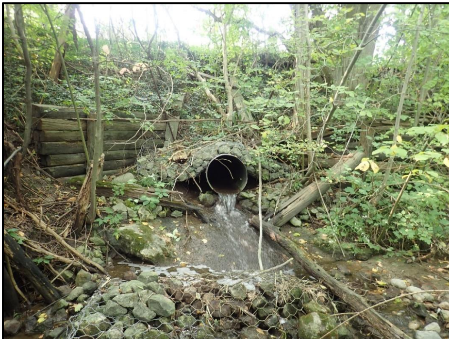
Photograph 4. Tannery Creek West Tributary – Pond Outlet Pipe (September 16, 2020)
