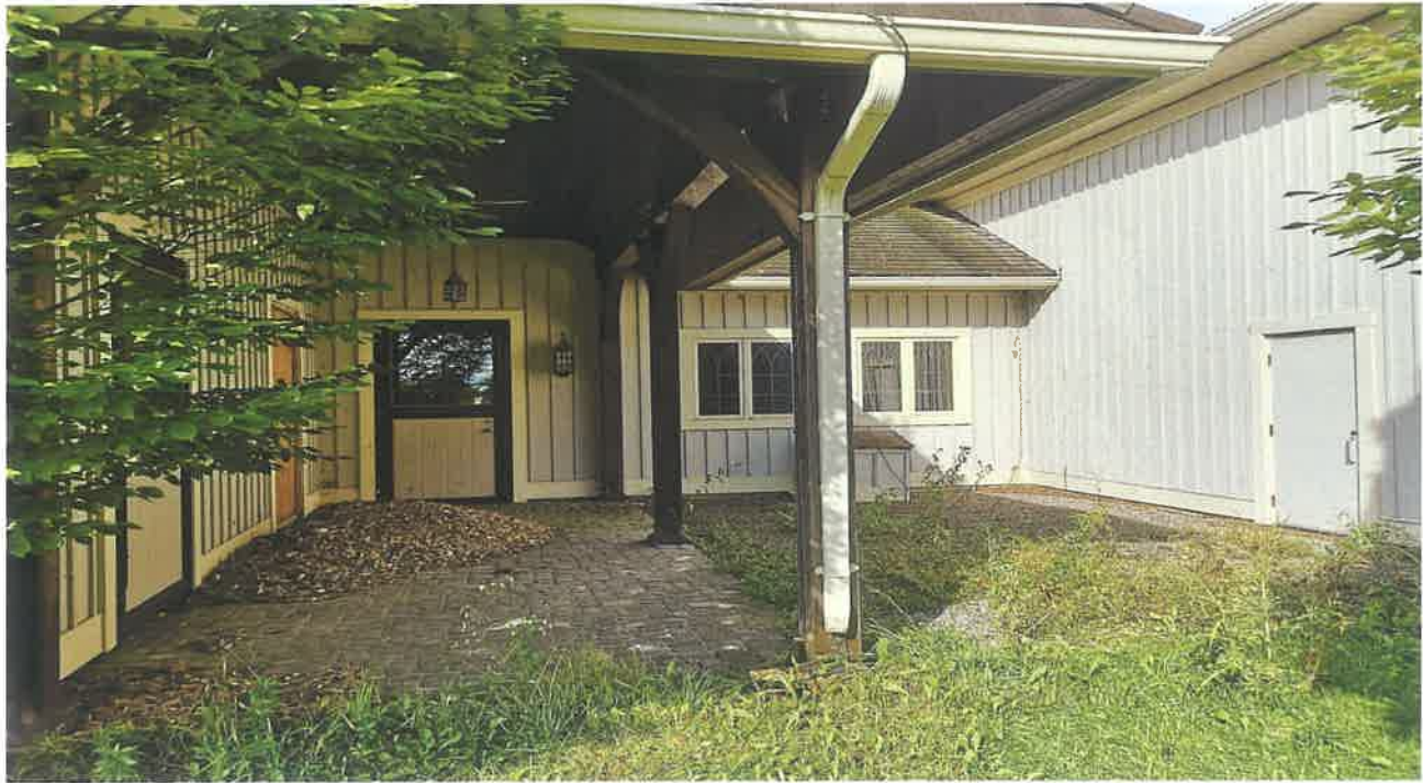
Stable at West portion of Subject Site (looking West)
