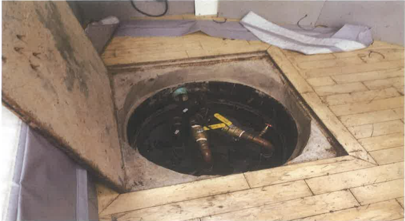
Sump Pit in Gym area of West Subject Site Residence
