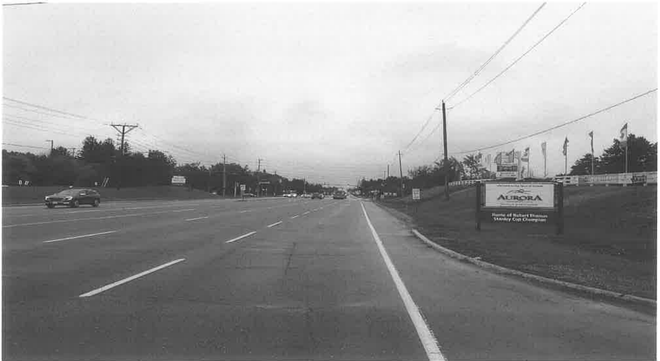
General view of Yonge Street (looking South)
