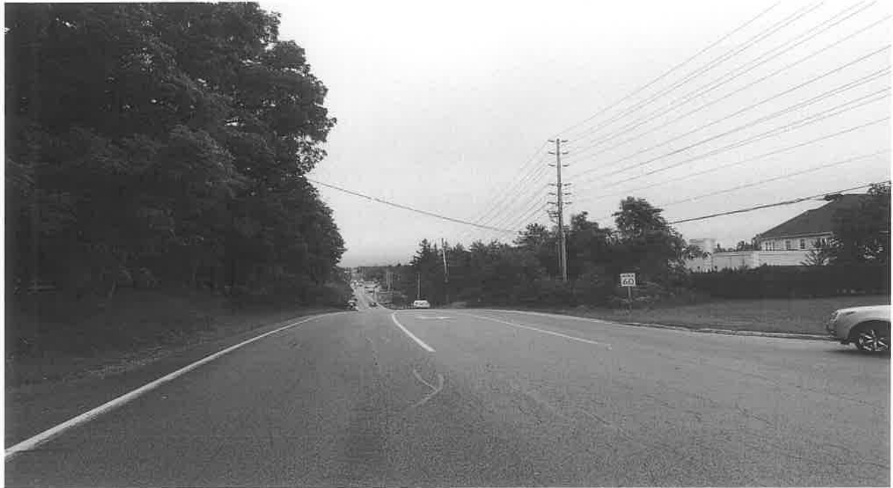
General view of St John's Sideroad (looking East)
