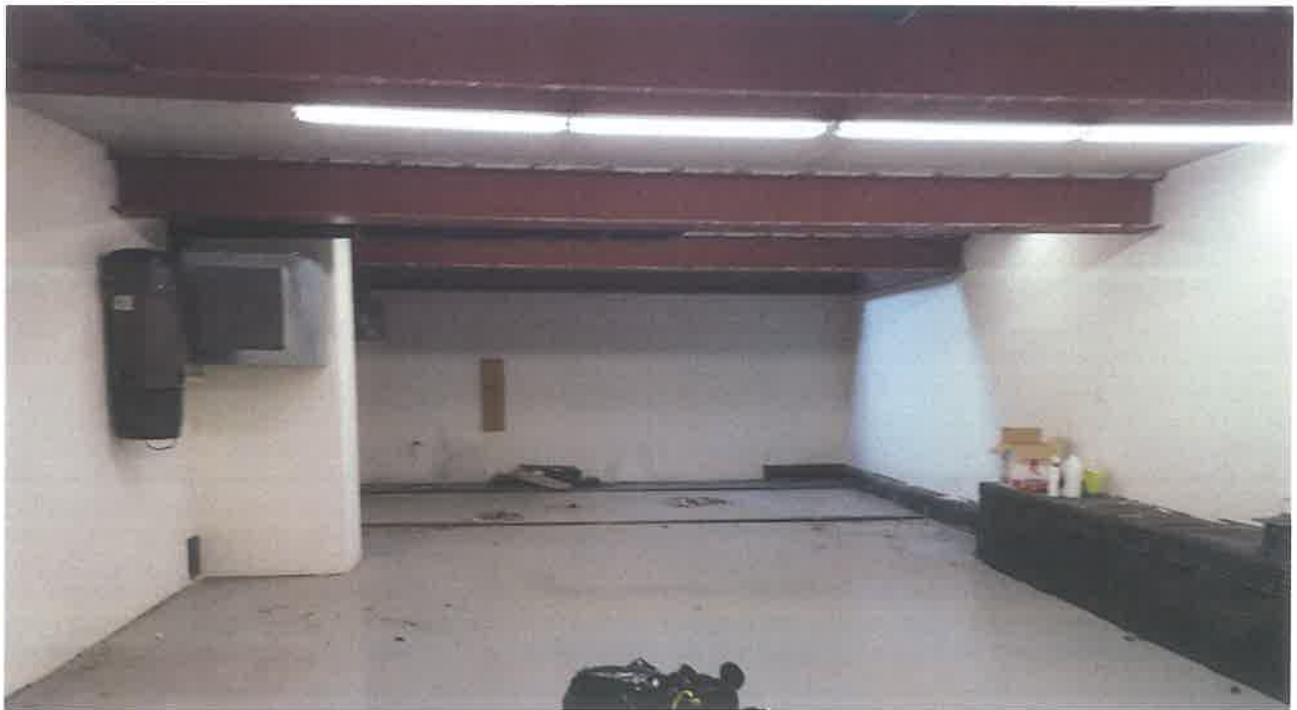
General View of Garage Basement
