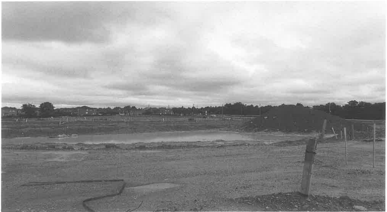
Construction area to North of Subject Site (looking North)
