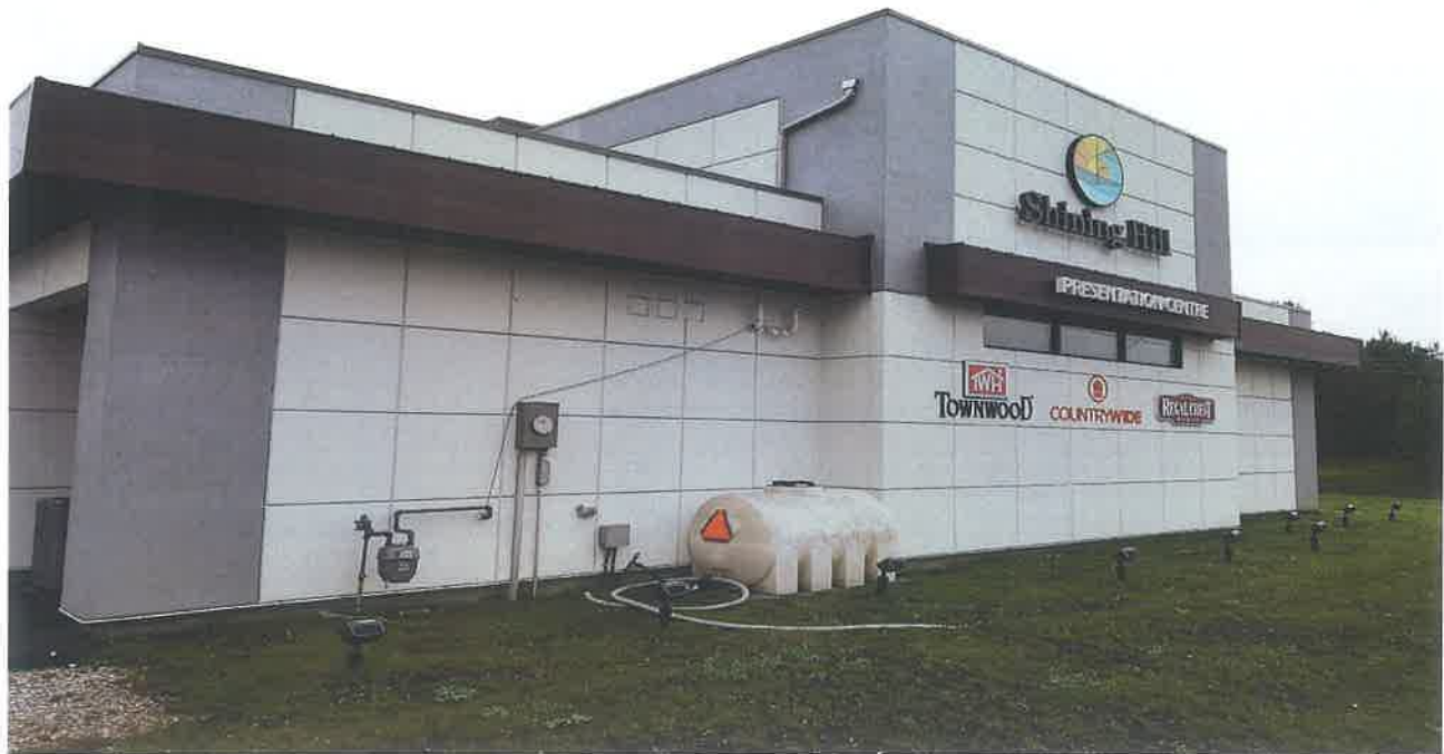
Sales Office near East boundary of Subject Site (looking West)
