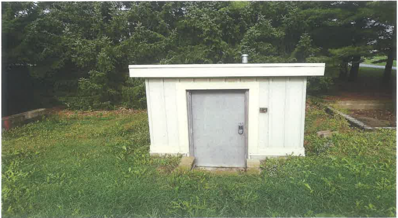
Utility Shed at West portion of Subject Site
