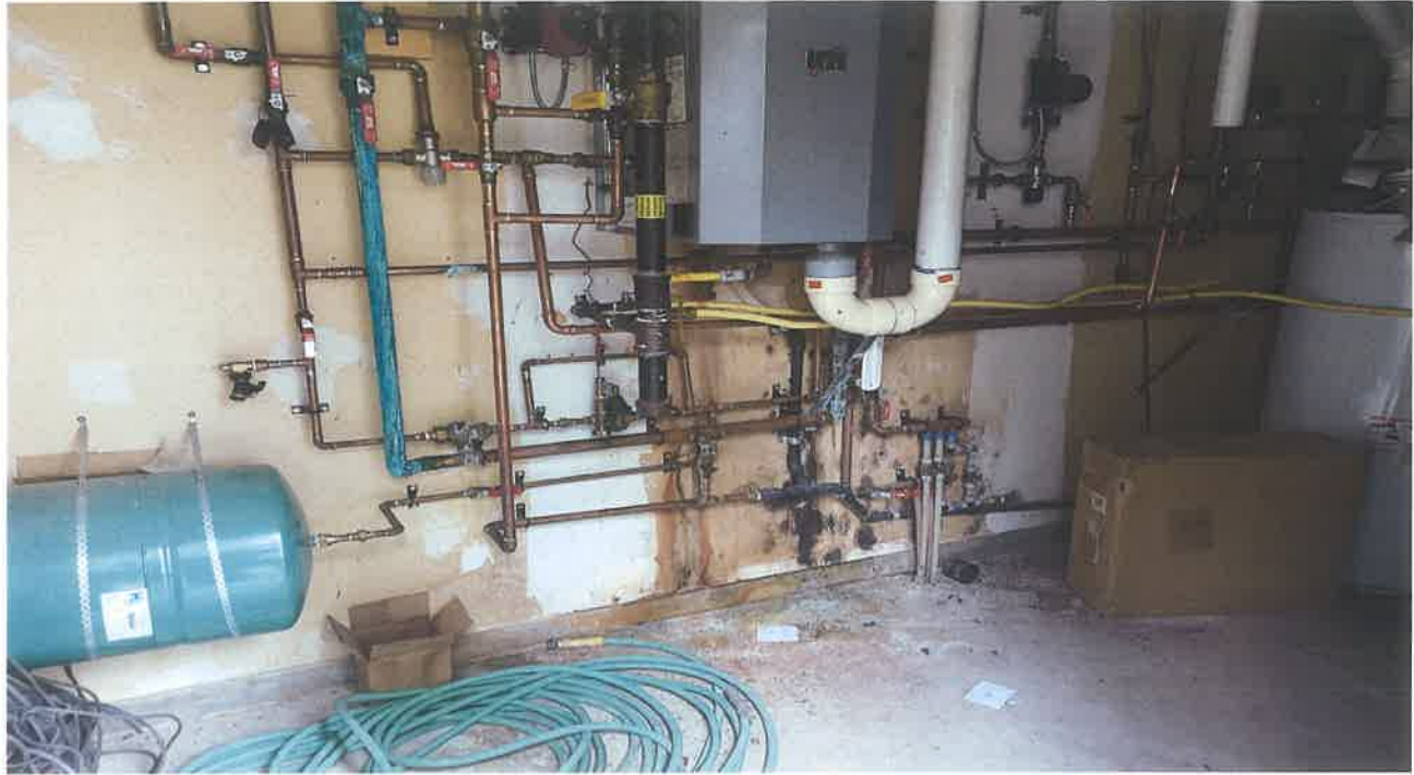
Utility room of Stable at West portion of Subject Site
