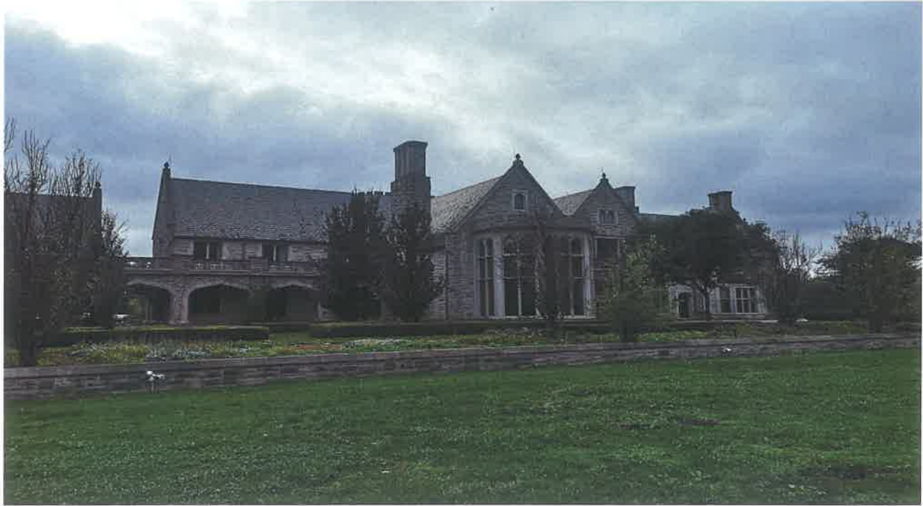
General view of West Subject Site Residence (looking South)
