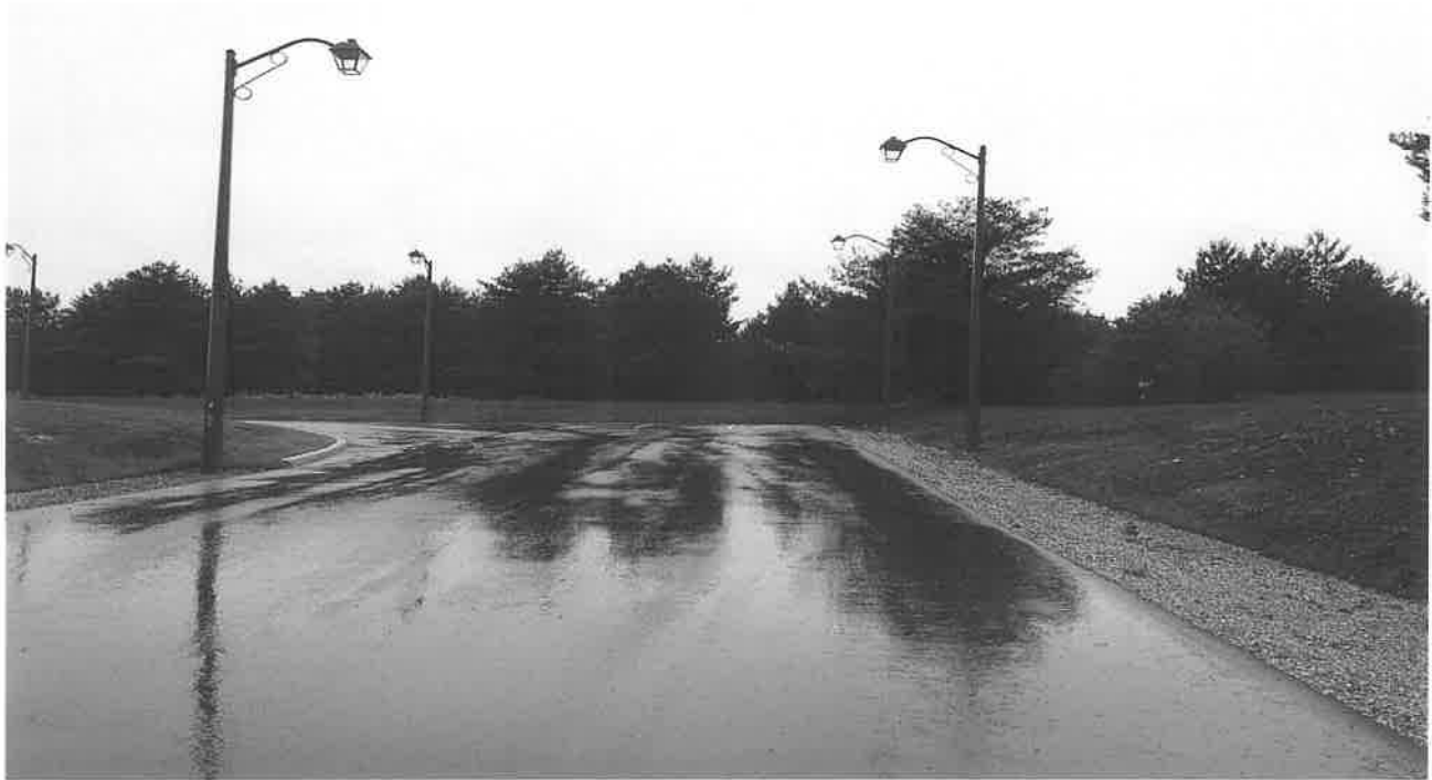
Gated entrance to Sales Office near East boundary of Subject Site (looking West)
