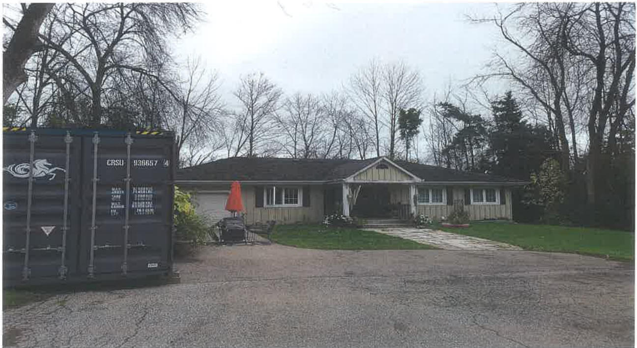
Residence at East portion of Subject Site (looking East)
