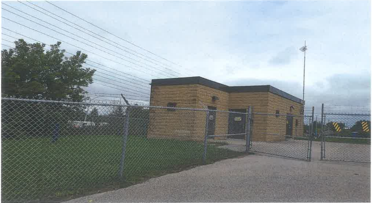
Water Treatment Facility to East of Subject Site (looking East)
