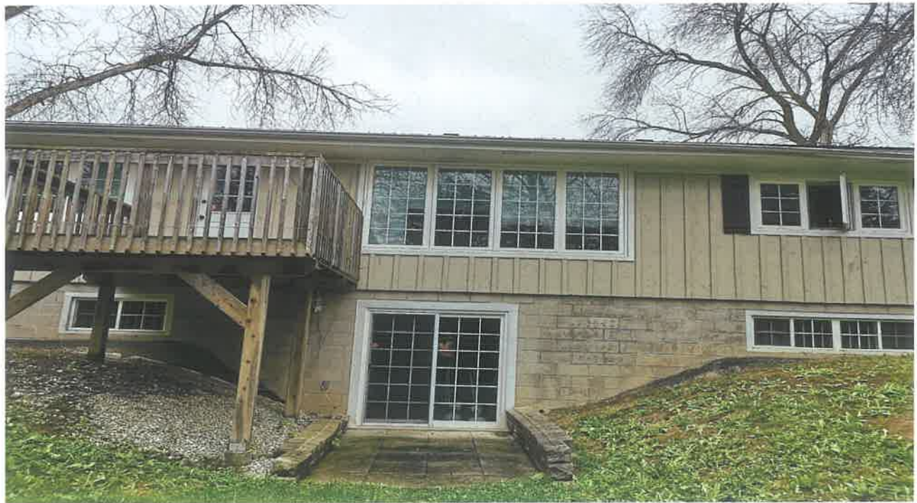
Residence at East portion of Subject Site (looking West)
