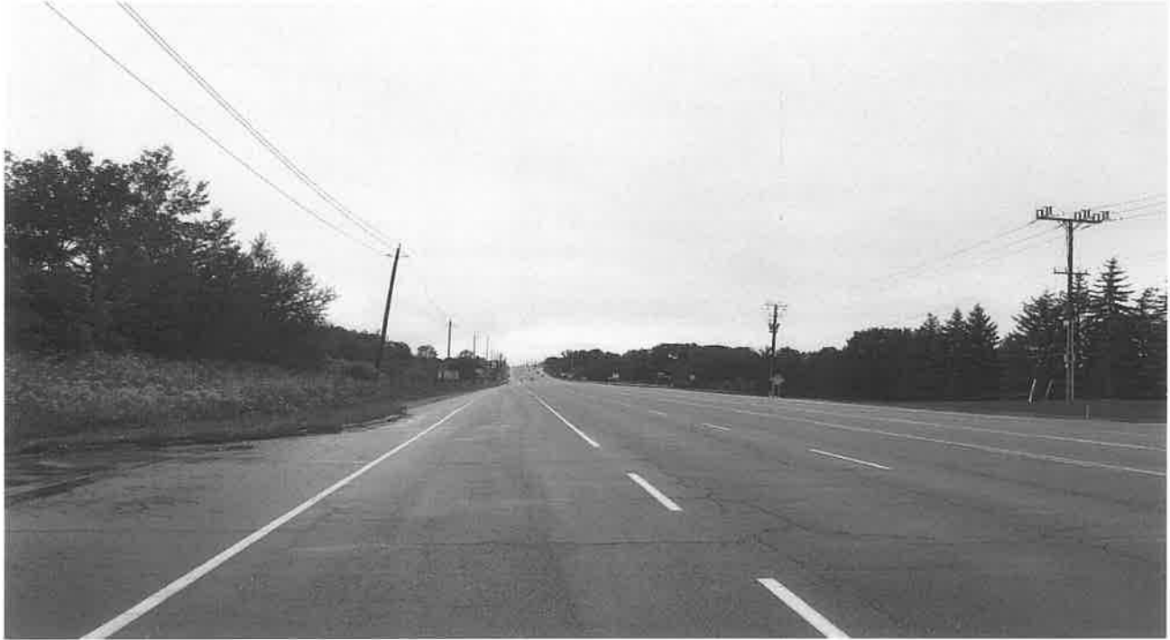
General view of Yonge Street (looking North)
