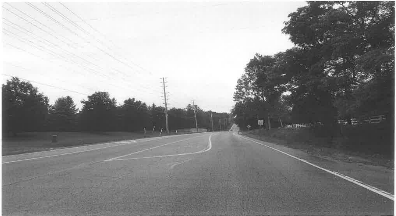
General view of St John's Sideroad (looking West)
