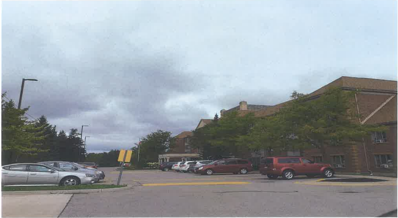
Apartment to East of Subject Site (looking North)
