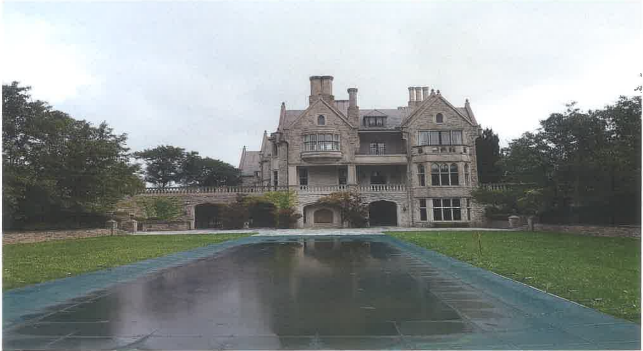
General view of West Subject Site Residence (looking Northeast)
