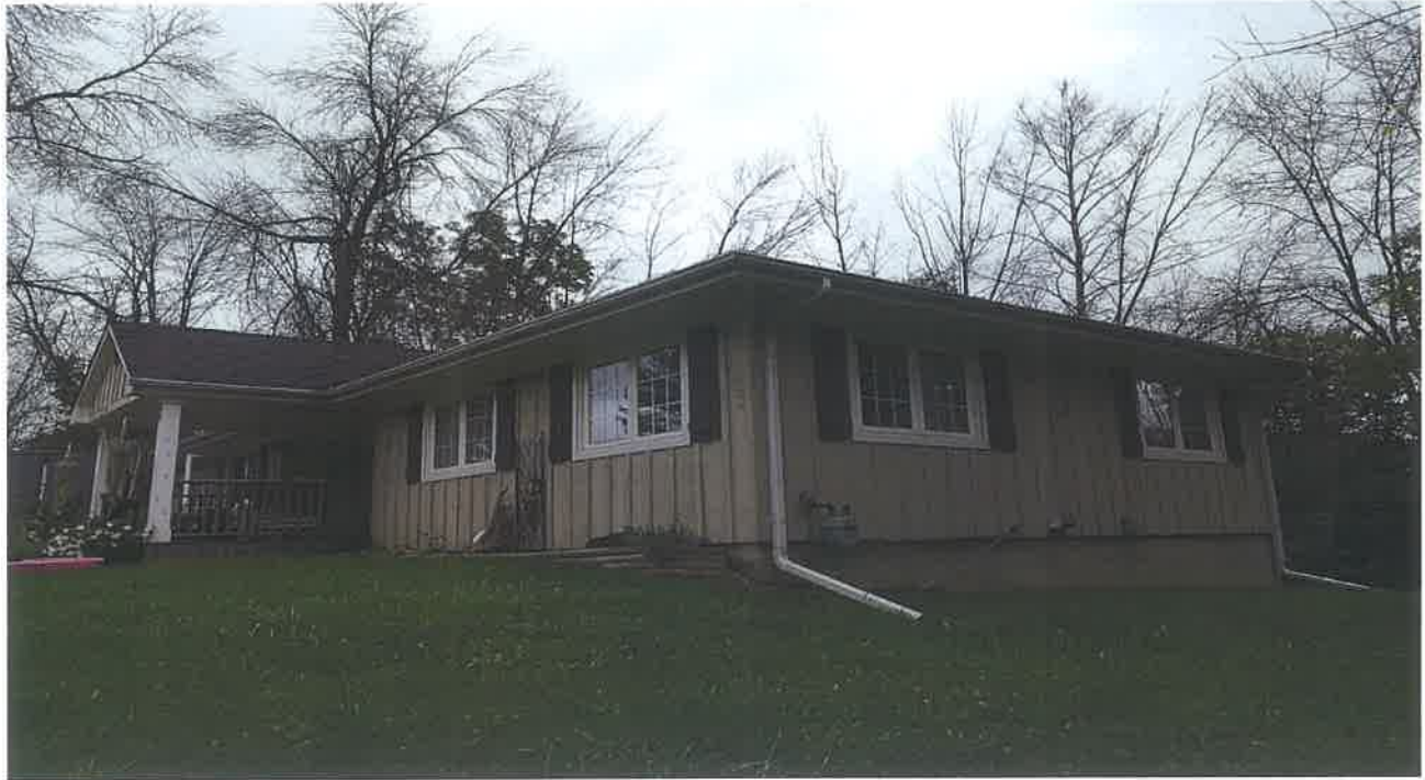
Residence at East portion of Subject Site (looking North)
