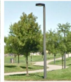
Lights - 15' pole height
