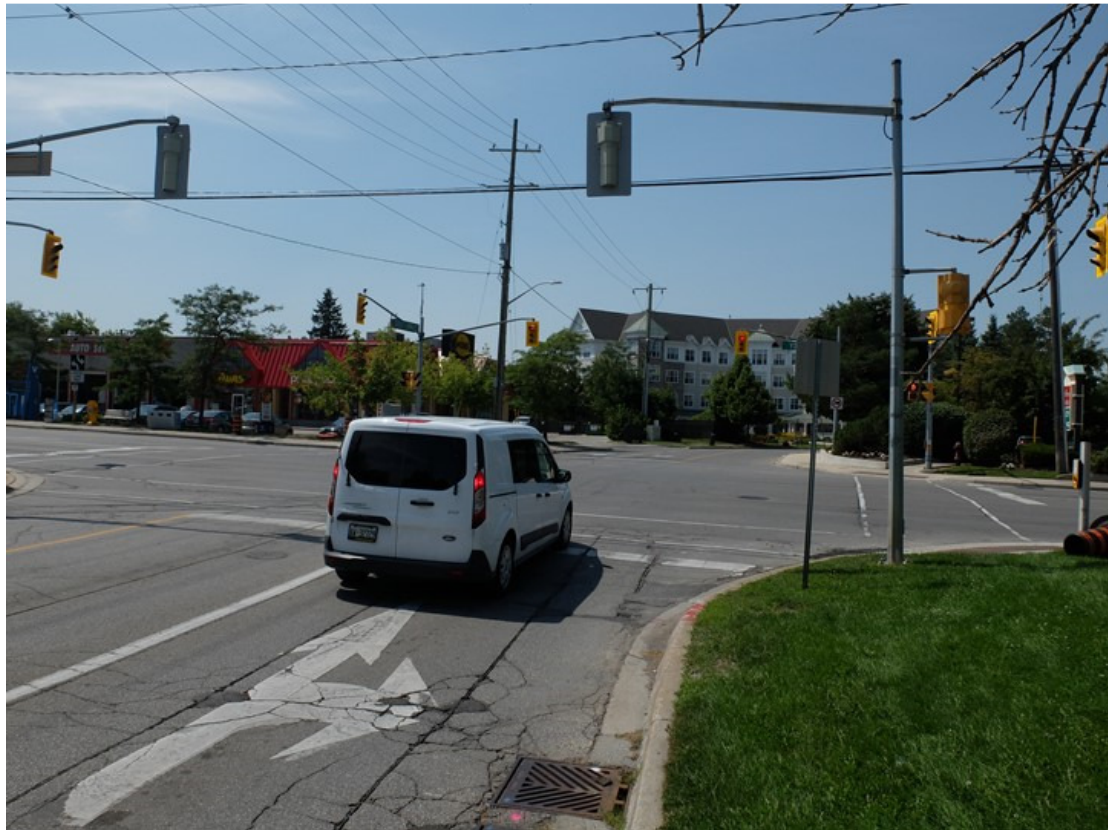
Figure 4-21: Yonge Street and Golf Links Drive/Dunning Avenue intersection
