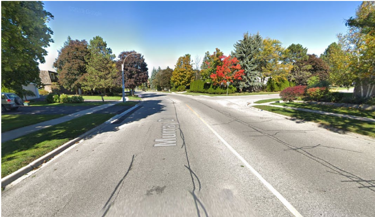
Figure 16: Existing Murray Drive ROW
