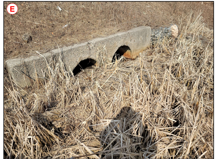
Existing Culvert Inlet Pipes and Headwall Structure
