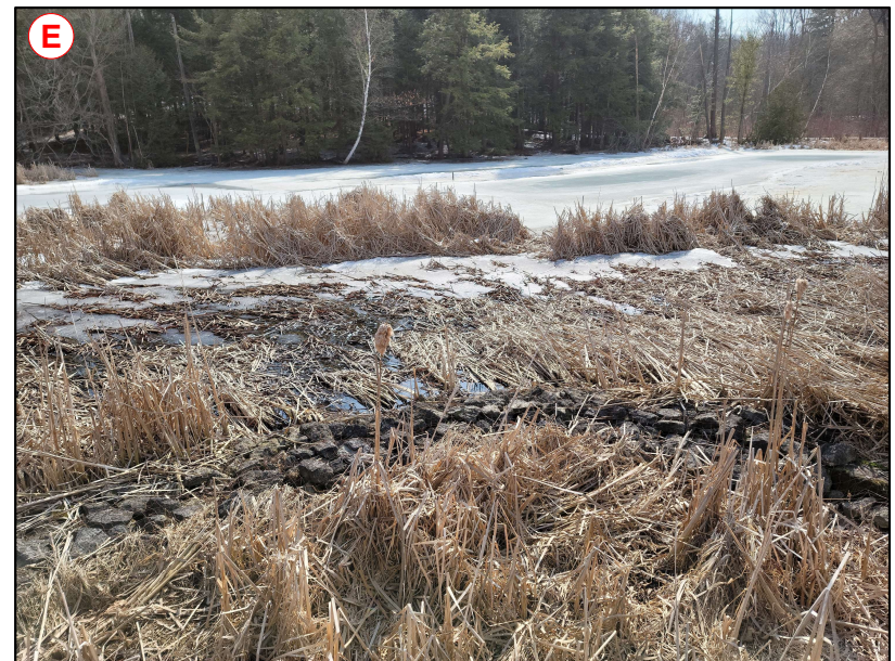
Salamander Pond Upstream of the Existing Culvert Inlet
