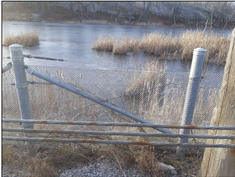
Example of Wildlife Fencing Installation with Steel Posts
