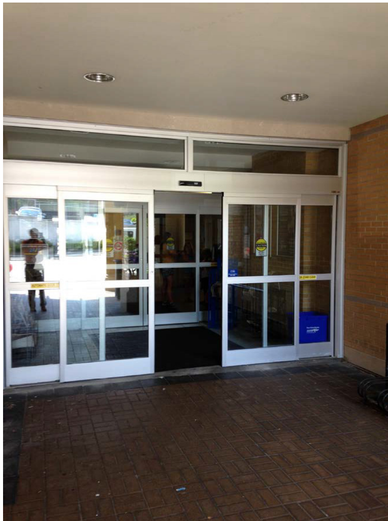
Barrier Free Sliding Glass Entrance at Aurora Public Library
