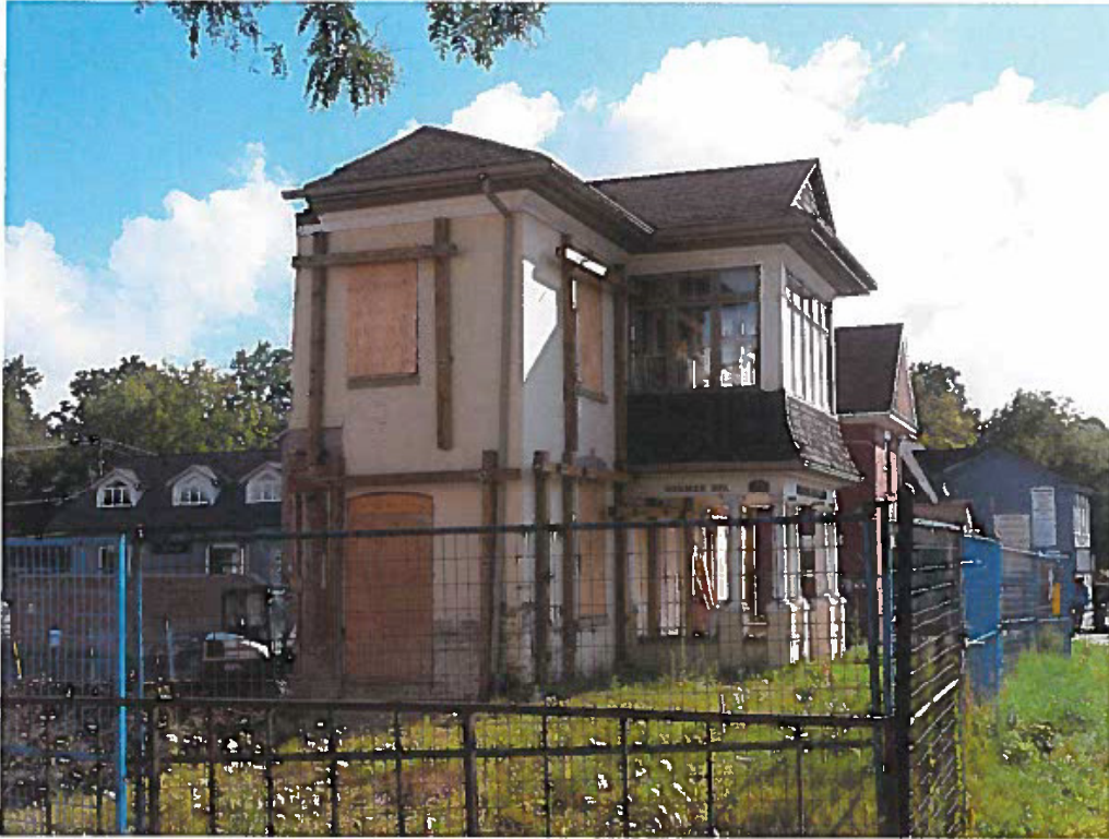
View of 32 Wellington Street East – South-West Elevation
