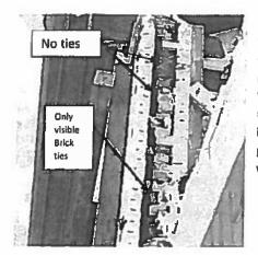
The existing load bearing veneer is in poor condition. The veneer is not adequately tied to act as load bearing masonry. The connection between the two (2) Inner Wythes is not continuous or solid. We are of the opinion that the wall does not meet the standards as a load bearing condition. As well, the outer façade is out of plumb because it is not adequately tied to the inward wall. Ties exceed the spacing of OBC Table 9.20.5.
