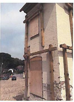
Picture #9 - Outer façade damage at west elevation
