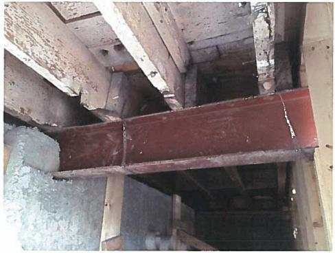
Picture #4 - Steel beam supporting ground floor framing
