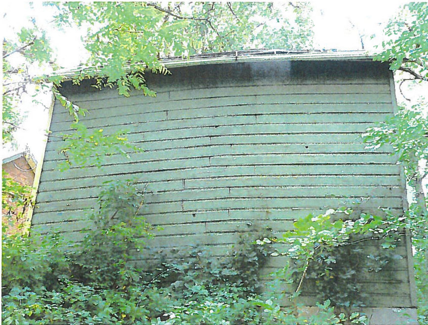
Existing Barn- Looking South
