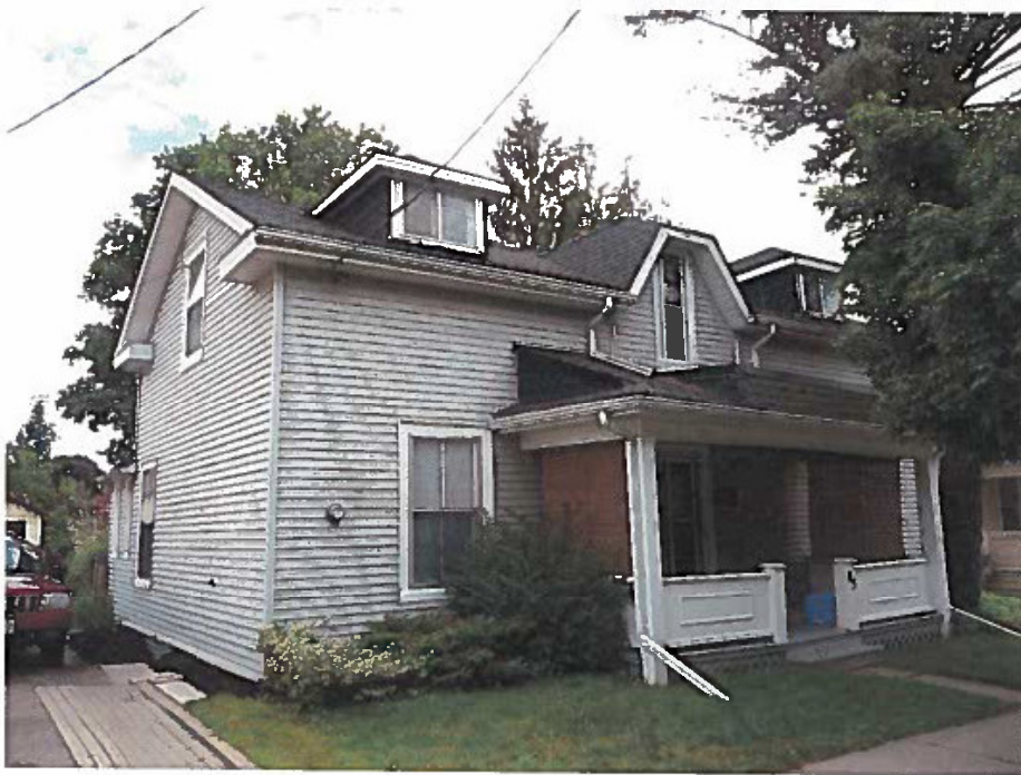
Existing Structure- Looking South
