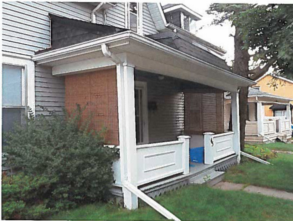
Existing Front Porch
