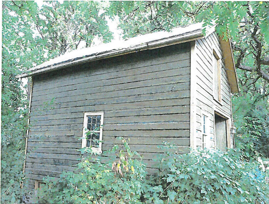
Existing Barn- Looking North-west
