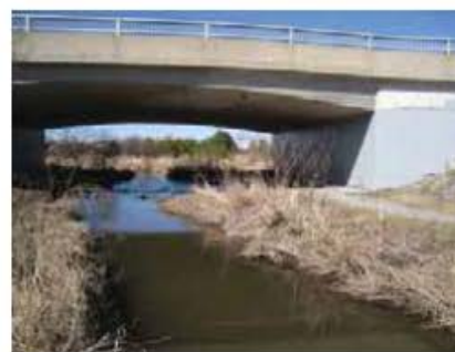
Trail Underpass, Aurora, ON
