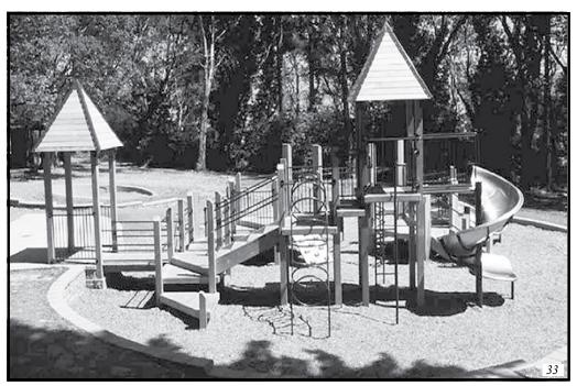
Accessible surfaces can include impact-attenuating tiles made of recycled rubber and engineered wood fiber that meet the ASTM requirements for accessibility and safety. The design can be created so safety is not compromised for individuals using the playspace where both standards are applied.
