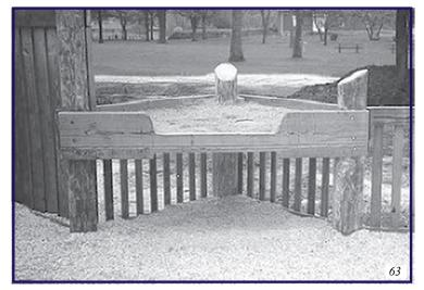
The edge of this elevated sand table has been designed to provide access by providing a generous opening. The tops of rims, curbs, or other obstructions that would prevent access to a table surface should be 787 mm (31.0 in) maximum in height.
