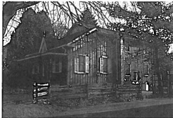
41 Metcalfe Street in December 2015
