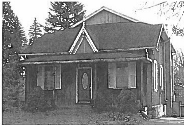
41 Metcalfe Street in December 2015
