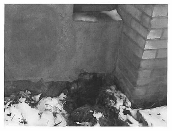
Photo 4. Loose foundation stones along the west side.
