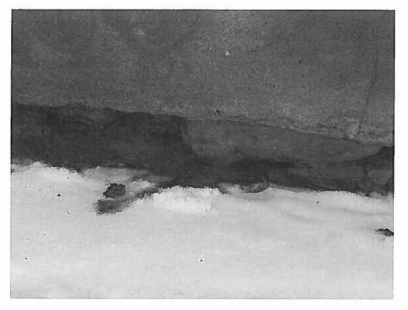
Photo 3. Deterioration of mortar along the west driveway.
