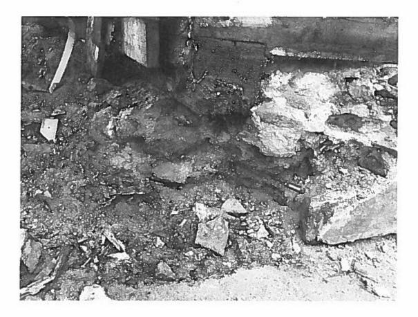
Photo 1. Failed foundation and deteriorated sill beam at north-west corner.
