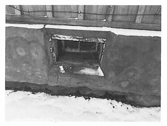
Photo 2. Deterioration of mortar along the west driveway.
