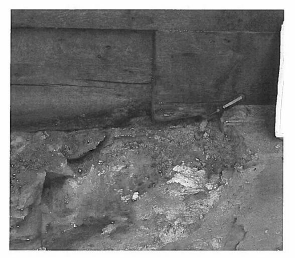
Photo 5. Deteriorated sill beam along the west foundation wall.
