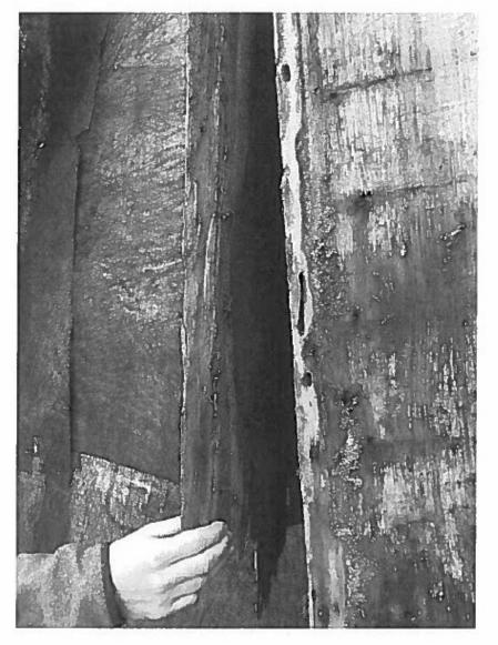
Photo 6. Evidence of carpenter ant activity in the walls above the sill beam (wood shavings and ant galleries.
