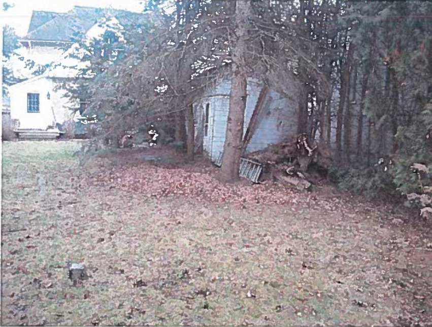
Rear view of existing attached shed, location of proposed garage to be located behind the existing accessory structure.
