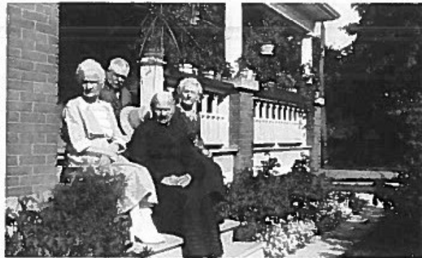
Thomas Cairns and unidentified ladies on front steps at number seven Kennedy Street West; no date. Part of the railing survives in 2016, or has been exactly reproduced. The verandah now extends only to the first column past the steps, allowing more light into the living room. Photo: from family tree "My Gillham/Cairns tree" by "Impkirby" at Ancestry.ca.
