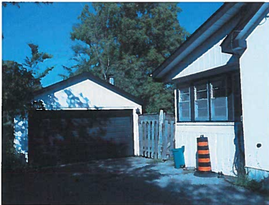
Accessory Structure- Looking West
