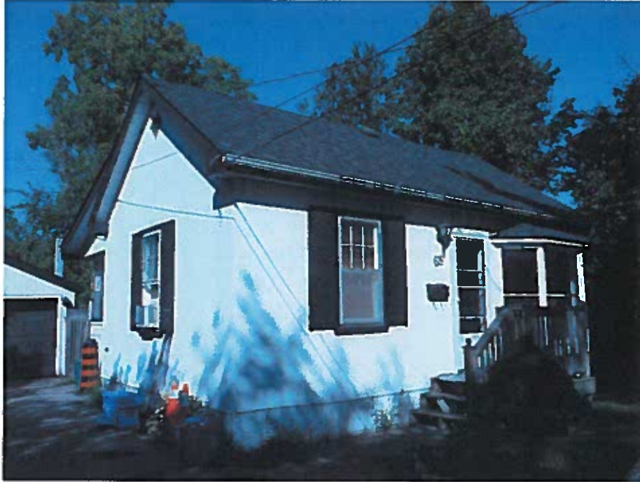
Front elevation- Looking West
