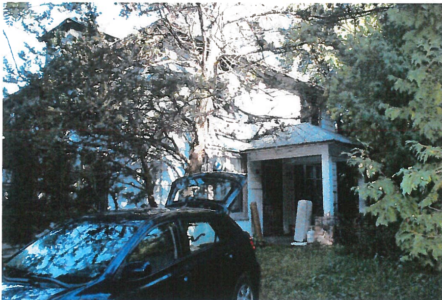
Side (north) elevation- Farmhouse
