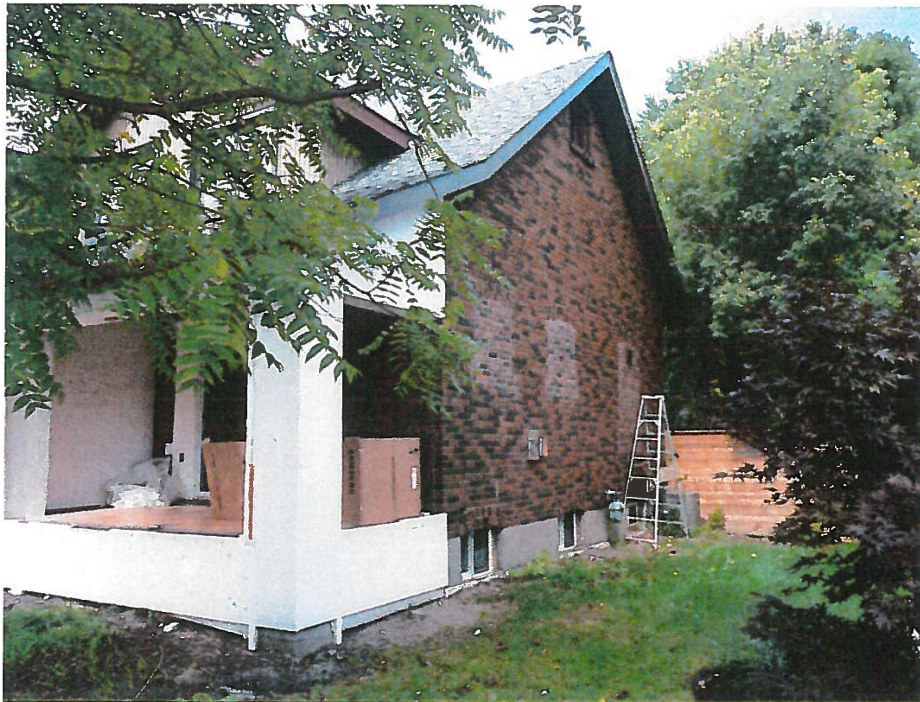
Side (east) elevation- Covered (bricked) window openings
