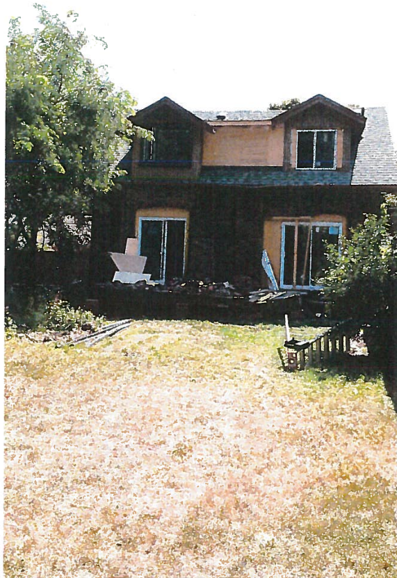
Rear Elevation- Modified roofline and two patio doors
