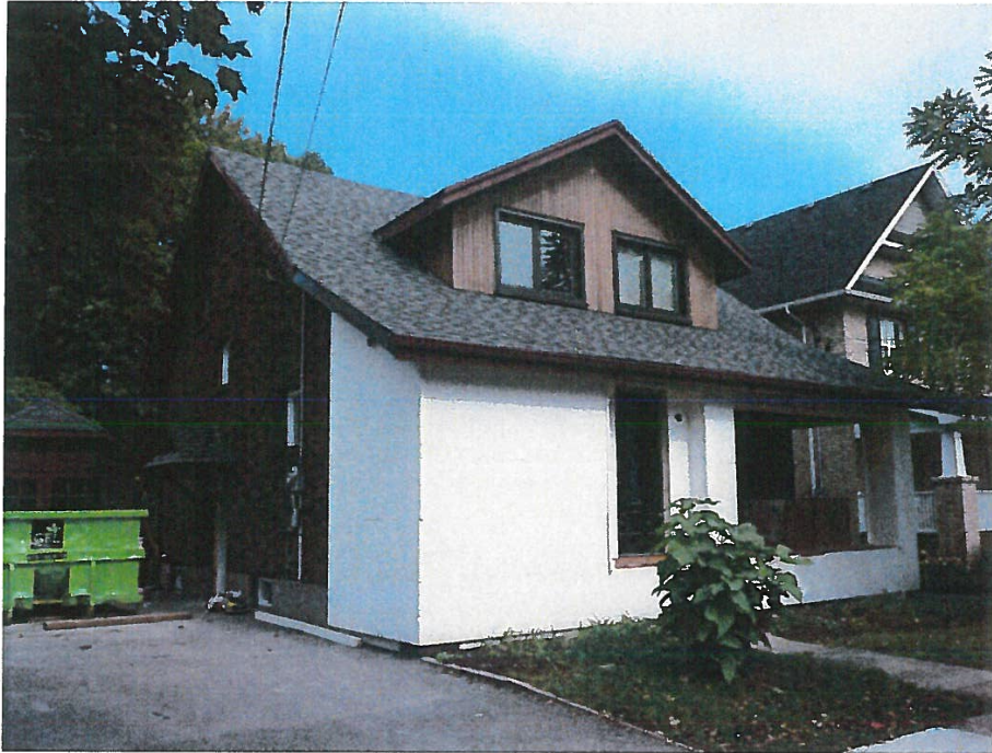
Front Elevation- Altered veranda and porch
