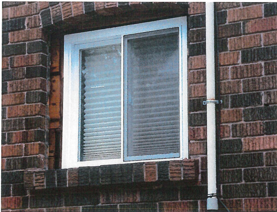
Side (west) elevation – Vinyl Windows
