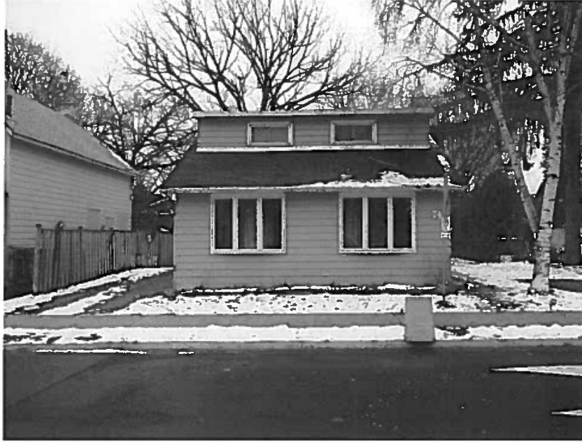
74 Centre Street- Front Elevation
