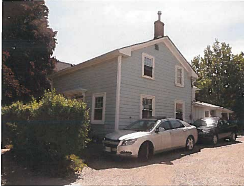
23 Mosley Street Front and Side (West) Elevation (Photo taken 2010).
