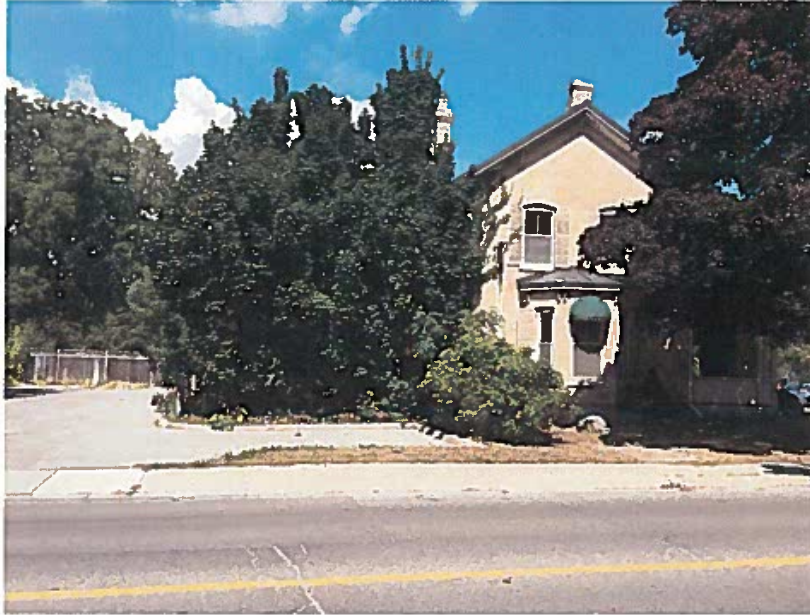
15032 Yonge Street - South Elevation. Addition proposed to be demolished is hidden behind existing trees
