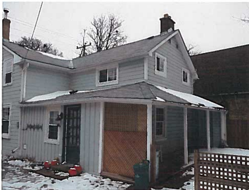
23 Mosley Street- Existing rear addition proposed to be removed
