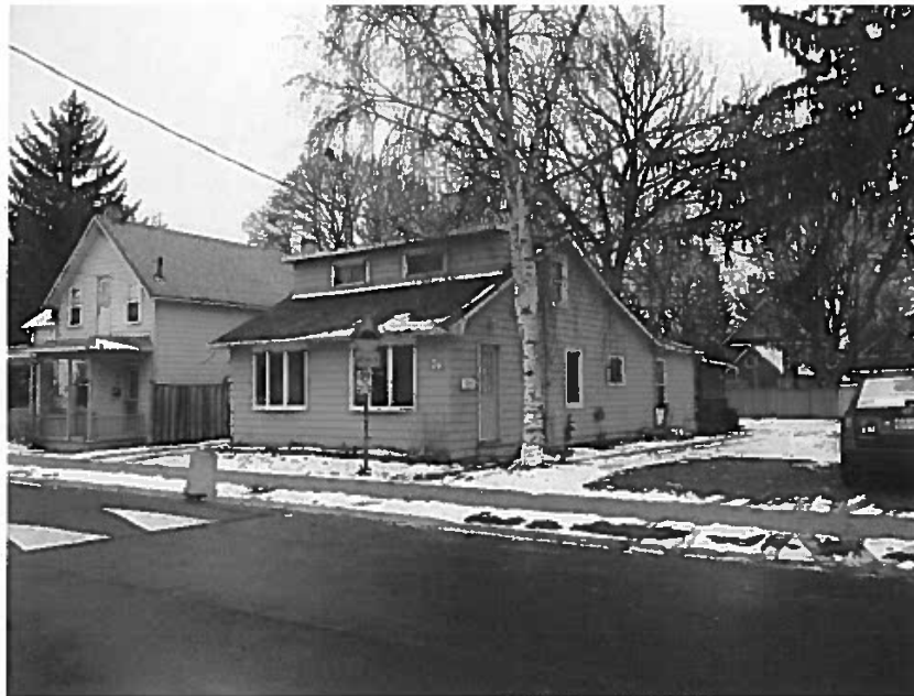
74 Centre Street- Front Elevation and East Elevation
