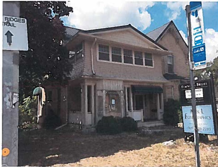
15032 Yonge Street – Front Elevation (looking northwest).
