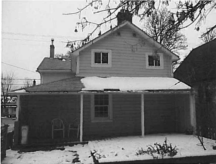
23 Mosley Street- Existing rear addition proposed to be removed
