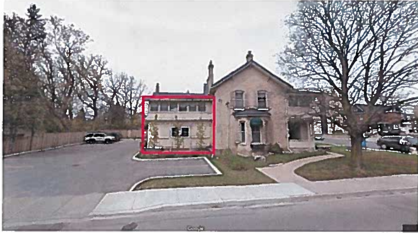
15032 Yonge Street - South Elevation. Addition proposed to be demolished (shown in red outline), circa 2009.
