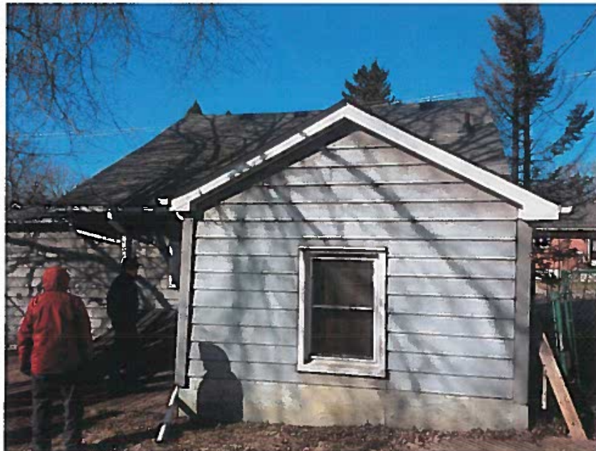
Rear elevation- Looking West
