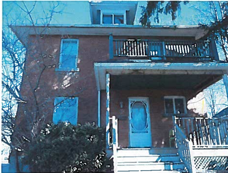
Front elevation- Looking North
