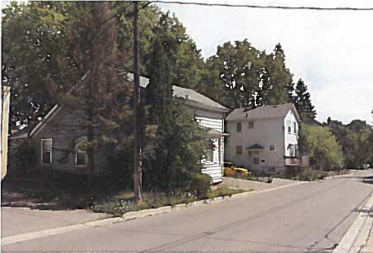
57 Temperance Street looking southeast with 55 Temperance in the foreground
