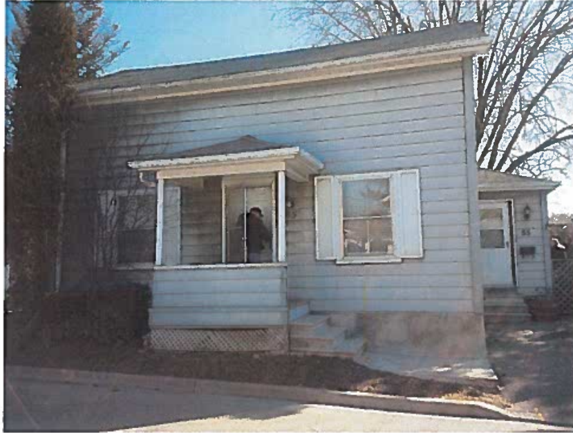
Front elevation- Looking East
