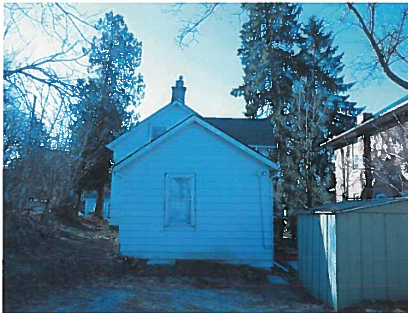
Rear elevation- Looking South
