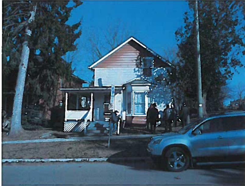
Front elevation- Looking North
