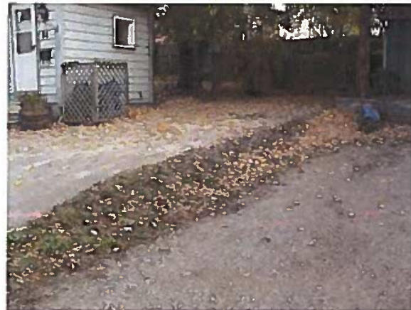
Plate 4: Difference in elevation between driveways of 55 (paved) and 57 Temperance Street (gravel), looking east-northeast (Photo DSC5811).
