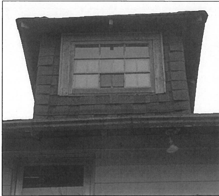
Figure 10: Above: South dormer with multipane sashes, plain trim, and asphalt shingle cladding, 2016. Stylistic exposed rafters are visible in the dormer and dwelling eaves.
