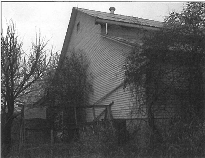
Figure 32: Left: South façade of barn, 2016.
