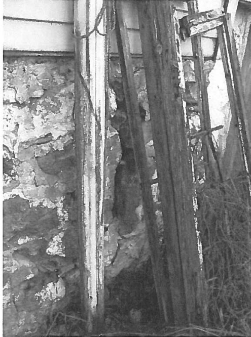
Barn #1, damaged rubble masonry wall
