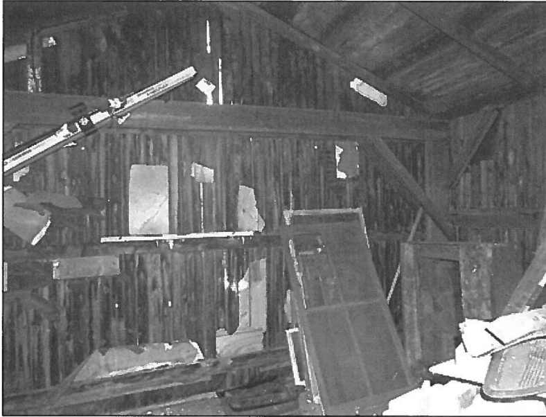
Figure 14: Above: Interior of summer kitchen/woodshed, 2016.
