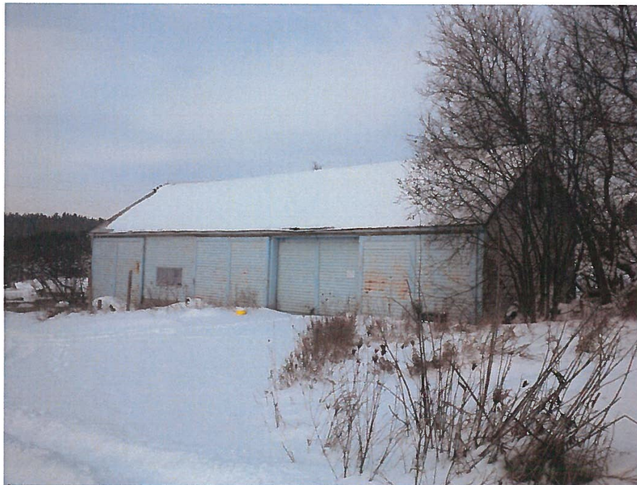
Existing Driveshed- looking Northwest
