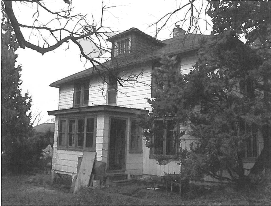
Farmhouse, south elevation
