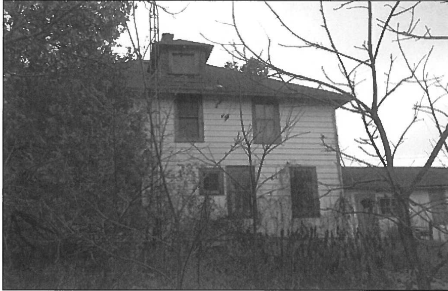
Figure 8: Above: North façade of house and summer kitchen/woodshed, 2016. Note the 2x2 panes type sash that differ from the east and south facades.
