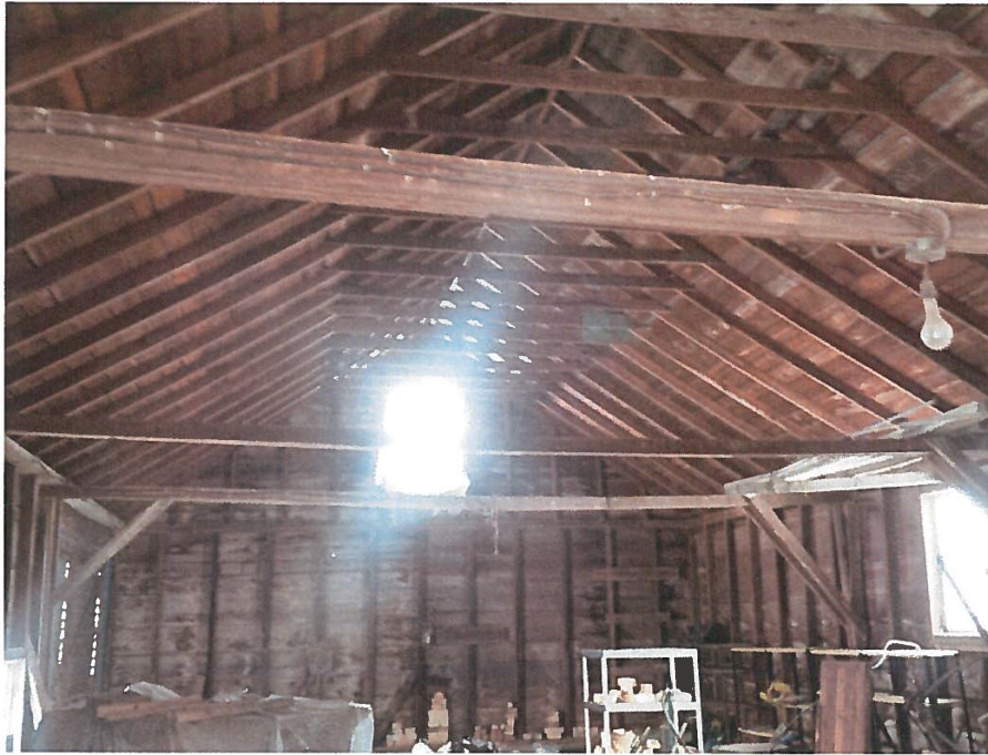
Interior of Driveshed
