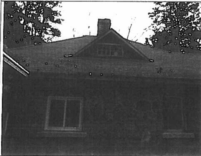
Plate 14: Windows, triangular dormer, and chimney on the west elevation, looking east
