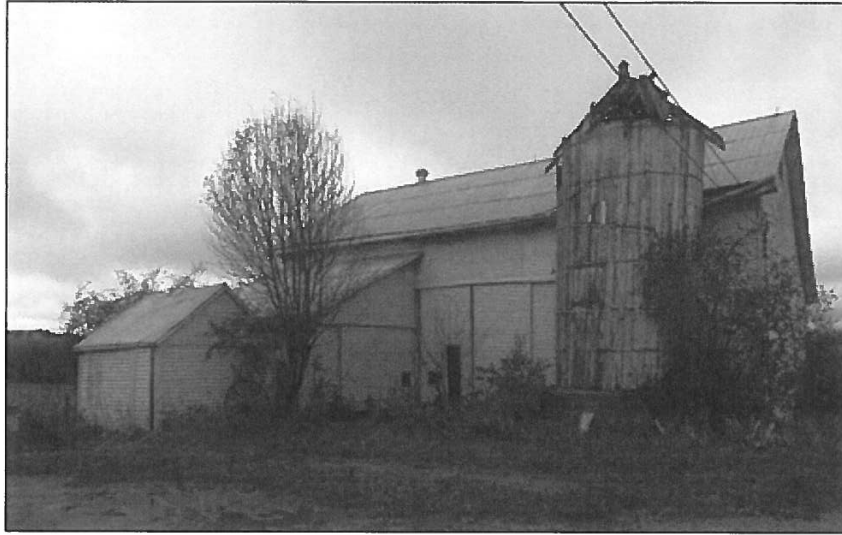
Figure 28: Above: East façade of larger east barn showing silo, shed roof addition, and standalone shed, 2016.
