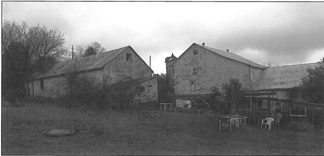
Figure 26: Looking southeast showing driveshed on left and barn complex on right, 2016.
