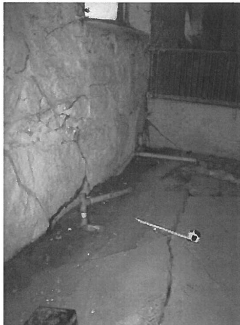
Barn #1, damaged rubble masonry wall
