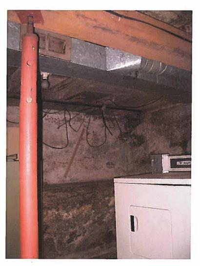
Basement showing support jack, spalling concrete, floor joist
