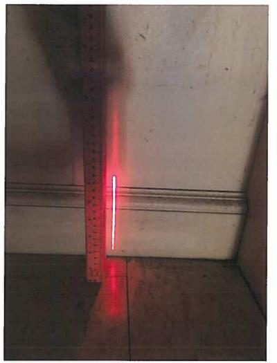
Close up showing degree of displacement in kitchen floor
