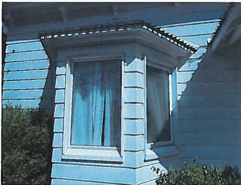
Figure 2- 16 Maple St, replaced windows
