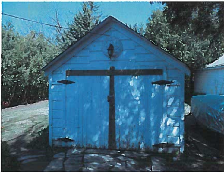
Figure 4- 16 Maple St, Existing Accessory Structure
