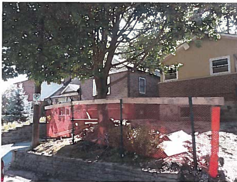
29 Mark- Front Elevation, Construction preparation ongoing. Existing Tree to be retained.
