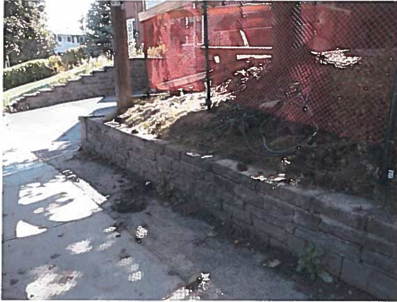
29 Mark- Existing Retaining Wall to be maintained.
