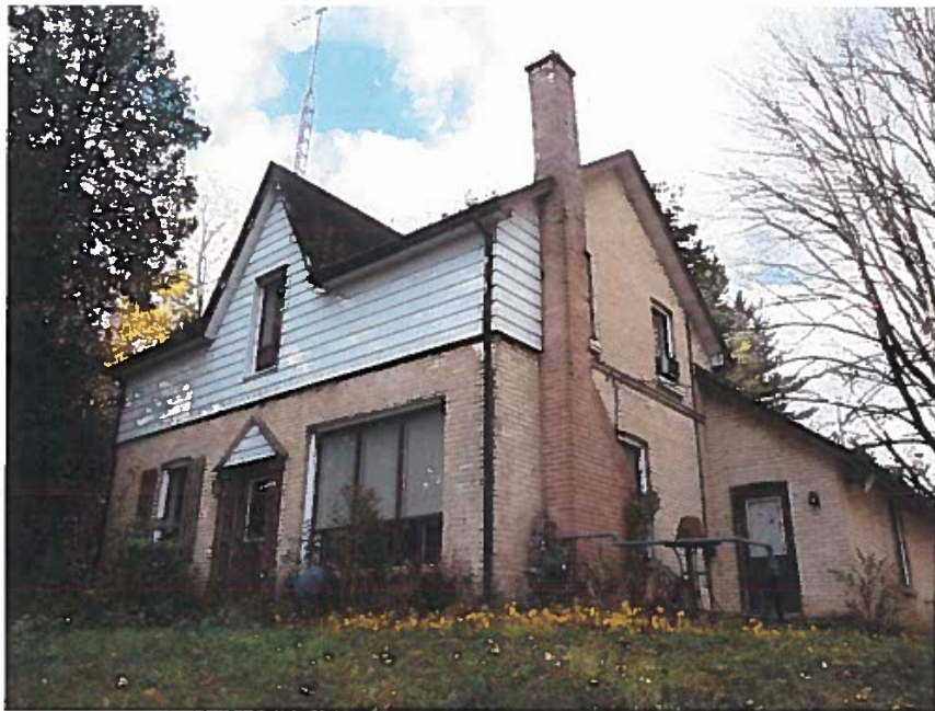
Cannon Farmhouse- Looking southwest
