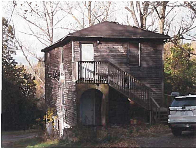
14288 Yonge Street- Second House constructed circa 1980
