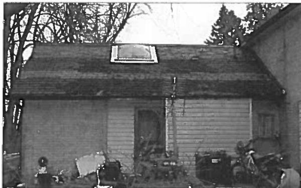
Figure 8 south facade - summer kitchen wing, aluminum siding
