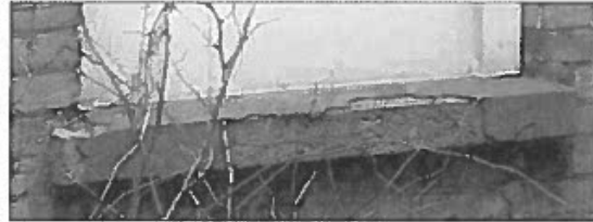
Figure 14 rendered concrete sill
