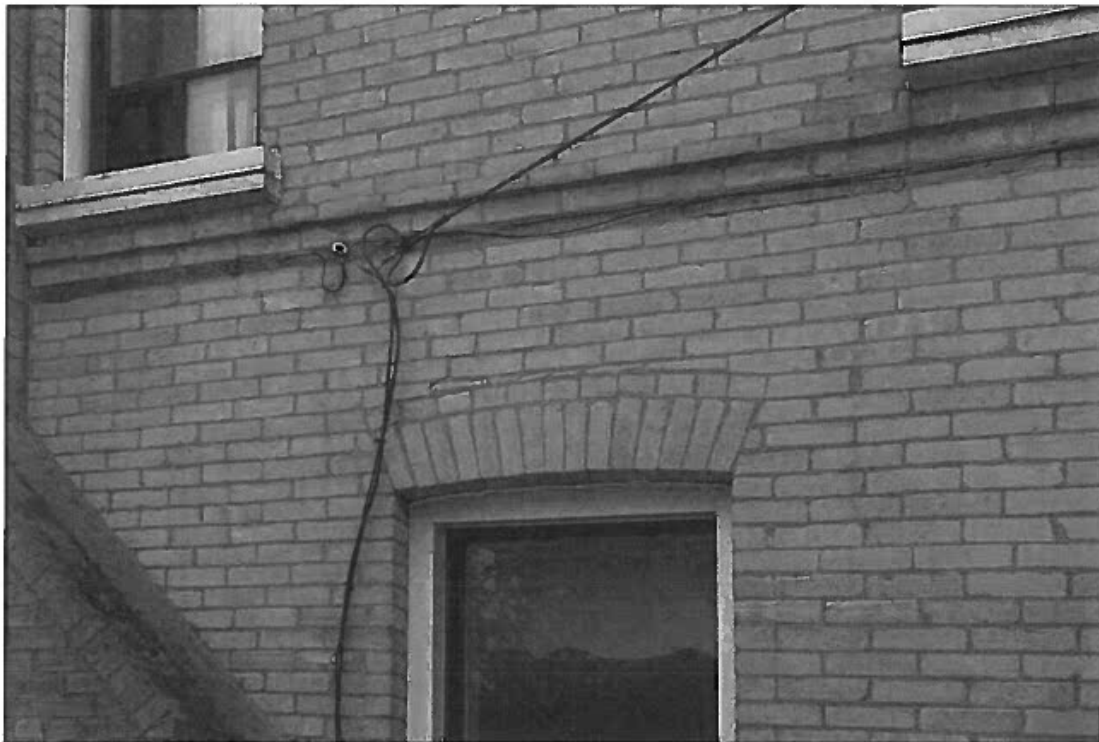
Figure 15 string course on north wall, aluminum clad sills and window frames
