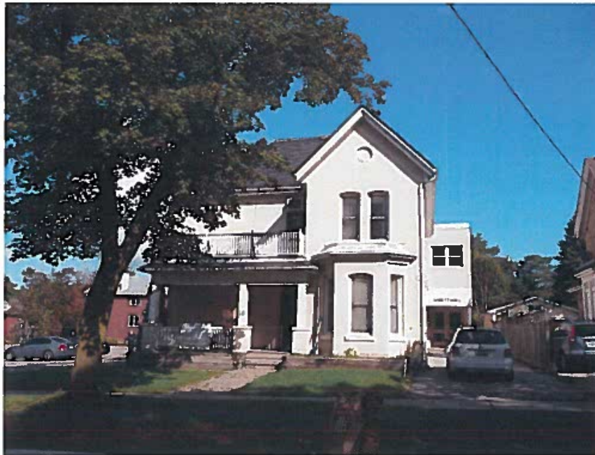
16 Catherine Avenue looking north from Catherine Avenue (September 2017)
