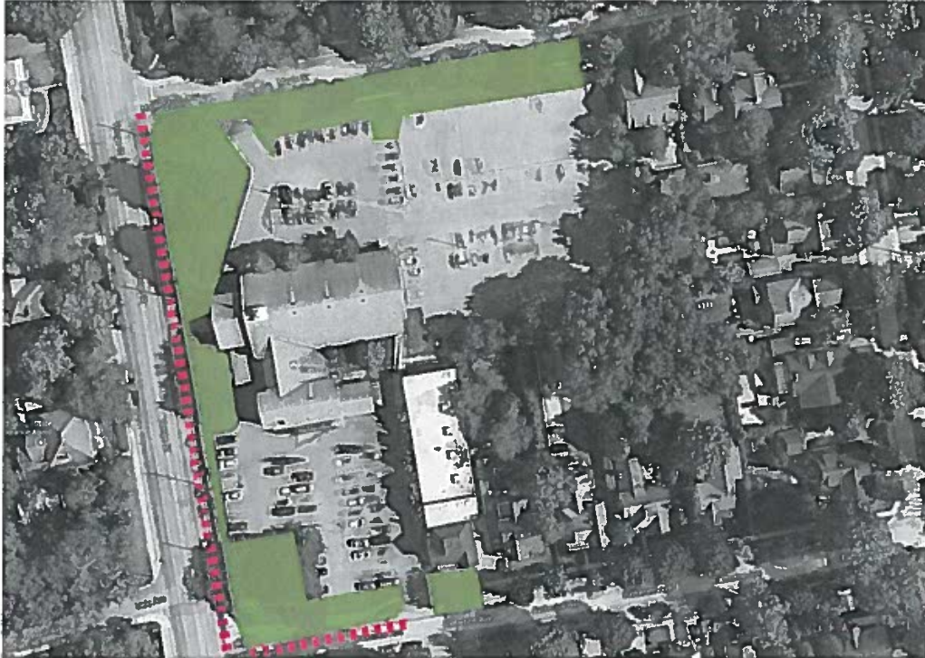
Aerial photograph annotated with elements of the Site that contribute to the character of the HCD (Google Maps, annotated by ERA).
