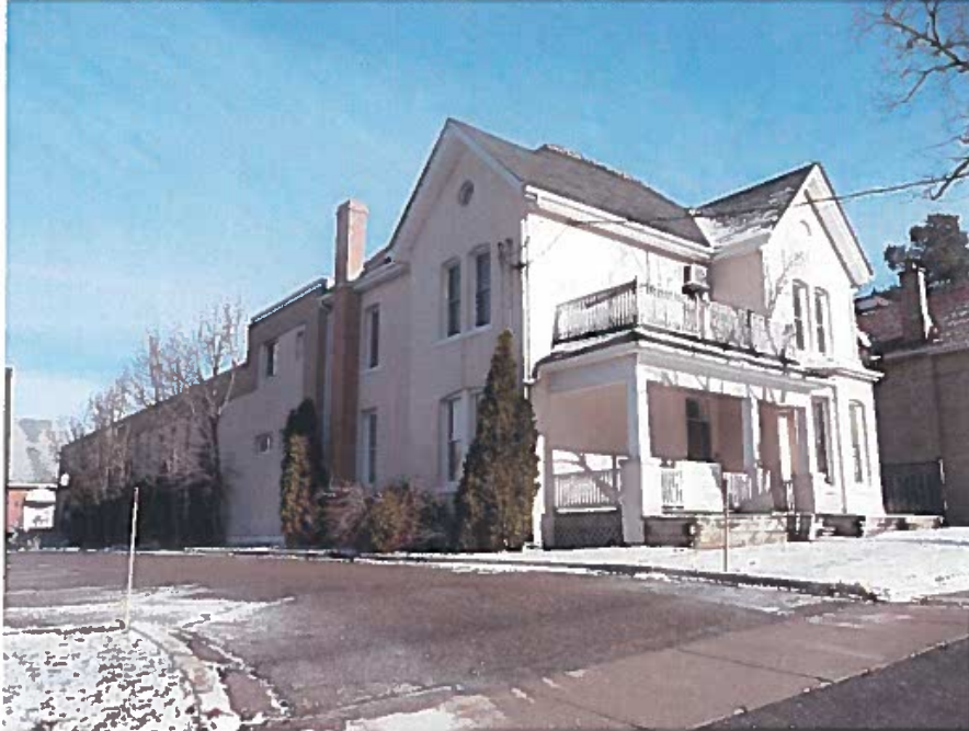
16 Catherine Avenue including Lynnet Hall looking northeast from Catherine Avenue
