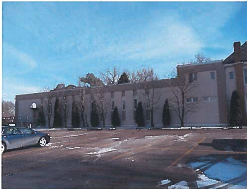
Lynnet Hall, proposed to be demolished- looking northeast from parking lot
