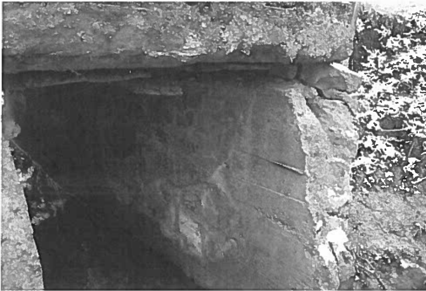
Plate 10: Detail of the concrete wall of the subject culvert.
