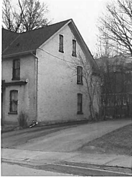
19-21 Machell Avenue – Side elevation (north), Photo 2018 Source: Town of Aurora
