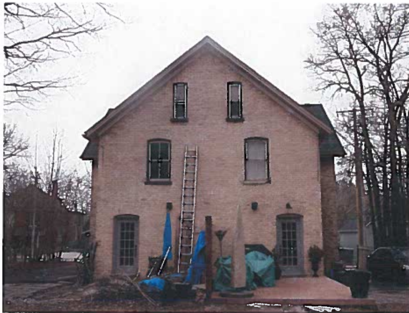
19-21 Machell Avenue – Rear elevation (west), Photo 2018 Source: Town of Aurora
