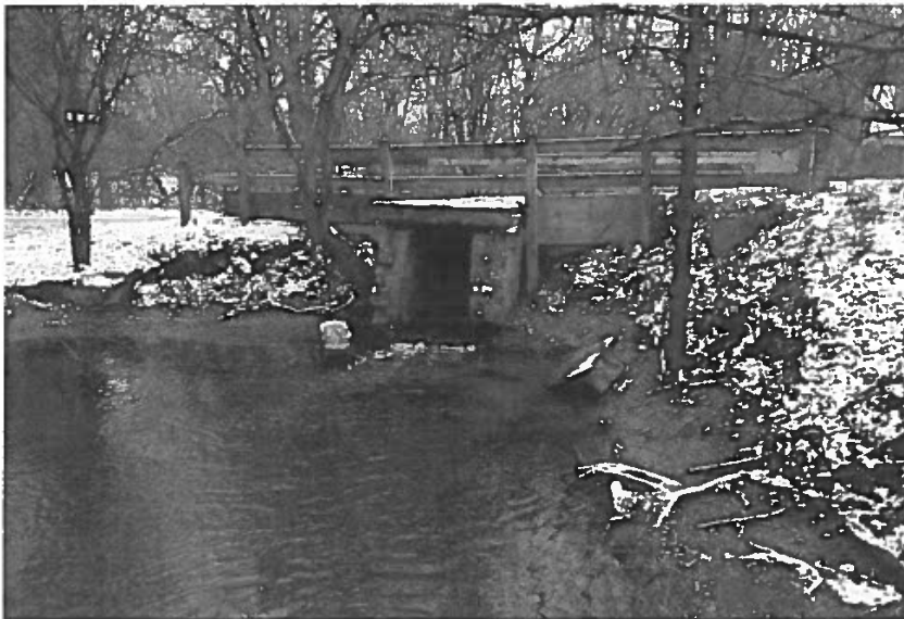
Plate 2: Looking south toward the subject culvert.
