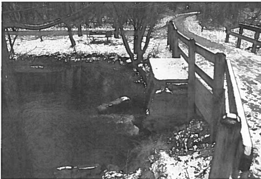
Plate 6: Oblique view of the north side of the culvert, looking east.
