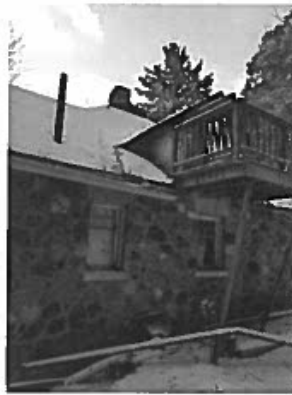
Photo#7: Second Floor Exterior Balcony ( general view )
