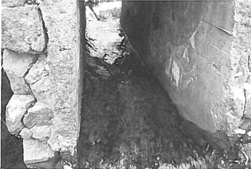
Plate 11: Detail of the watercourse running through the subject culvert.
