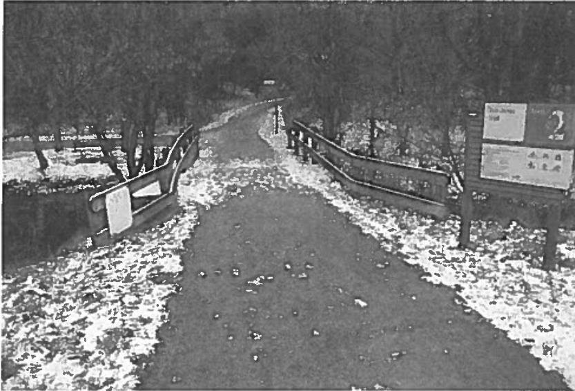
Plate 7 View along the pedestrian trail toward the subject culvert.
