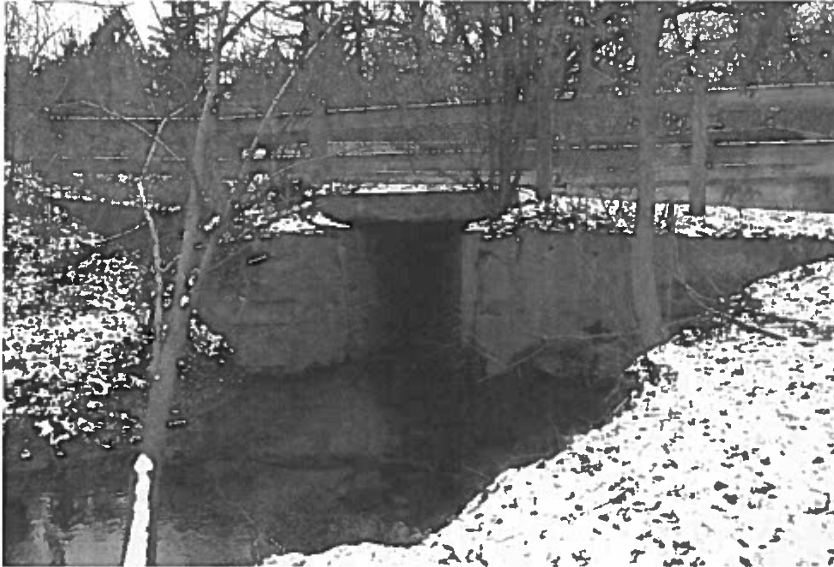
Plate 1: Looking north toward the subject culvert.
