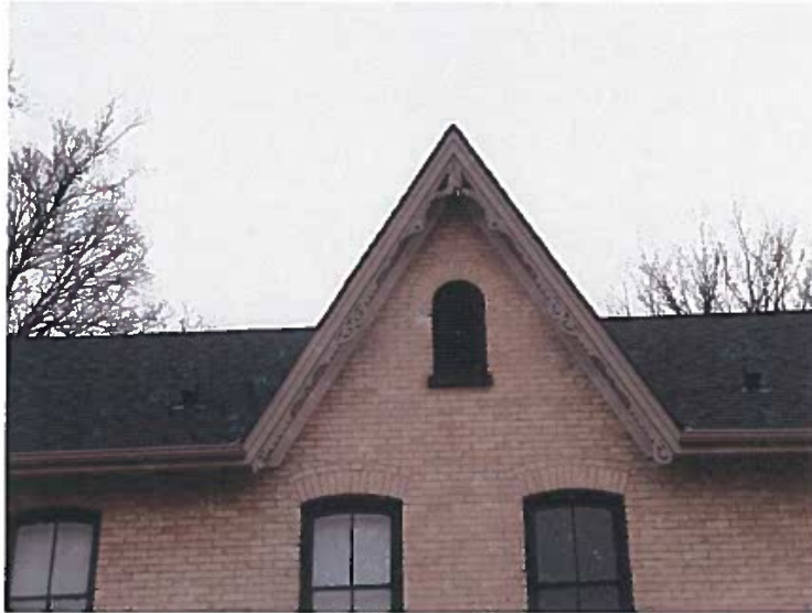
19-21 Machell Avenue –Gingerbread Bargeboard under centre gable - Photo 2018 Source: Town of Aurora
