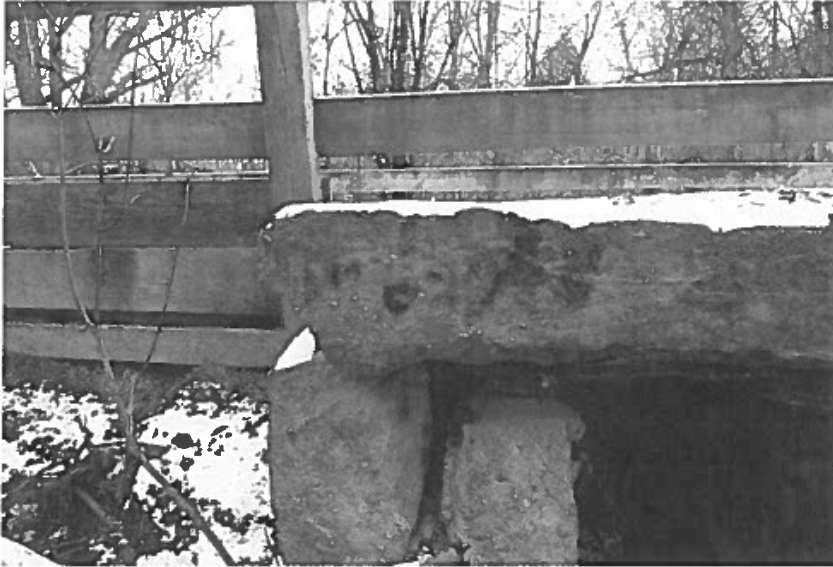
Plate 9: Detail of the concrete top of the subject culvert.
