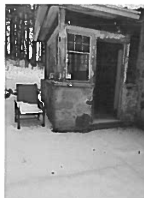
Photo #6 Back Entrance Vestibule (general view of door entrance)
