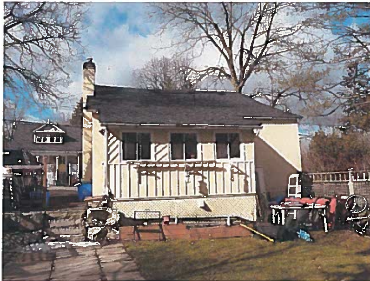
83 Temperance Street – Rear elevation, 1 storey rear addition not original to the home. Photo 2018 Source: Town of Aurora
