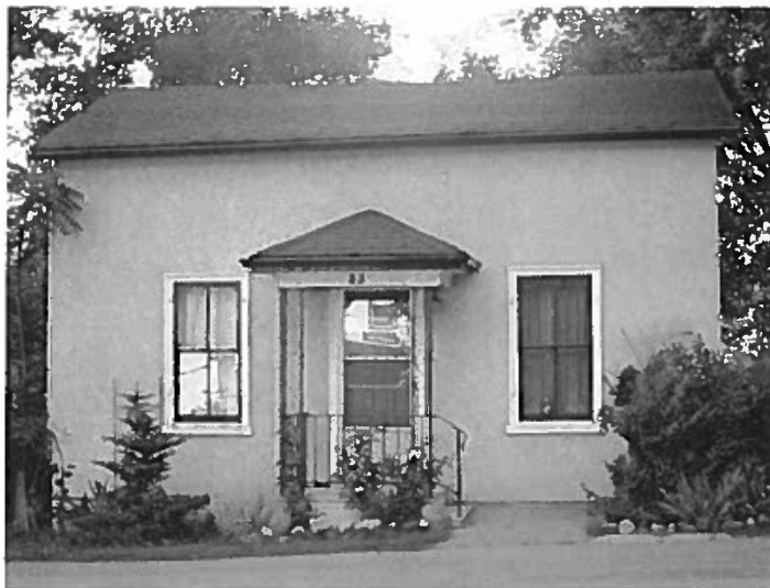
83 Temperance Street – Front elevation, Note the original 2 over 2 sash windows on the front elevation. Photo 1981 Source: Town of Aurora
