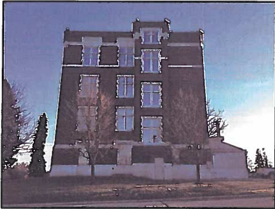
Image 16: North Elevation of former De La Salle College structure (November 27, 2017; View looking South)
