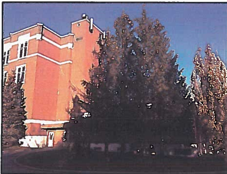
Image 13: Southwest corner of former De La Salle College structure and gymnasium addition (November 27, 2017; View looking Northeast)
