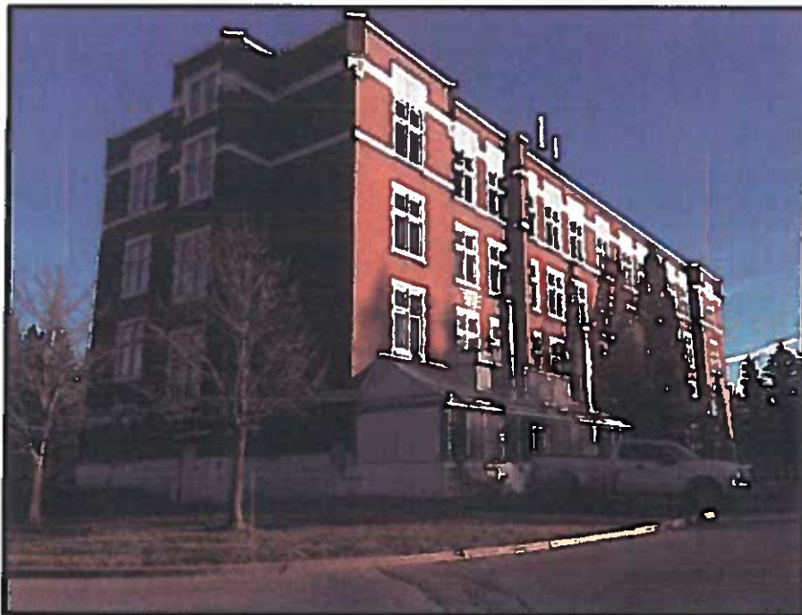
Image 15: Northwest corner of former De La Salle College structure (November 27, 2017; View looking Southeast)
