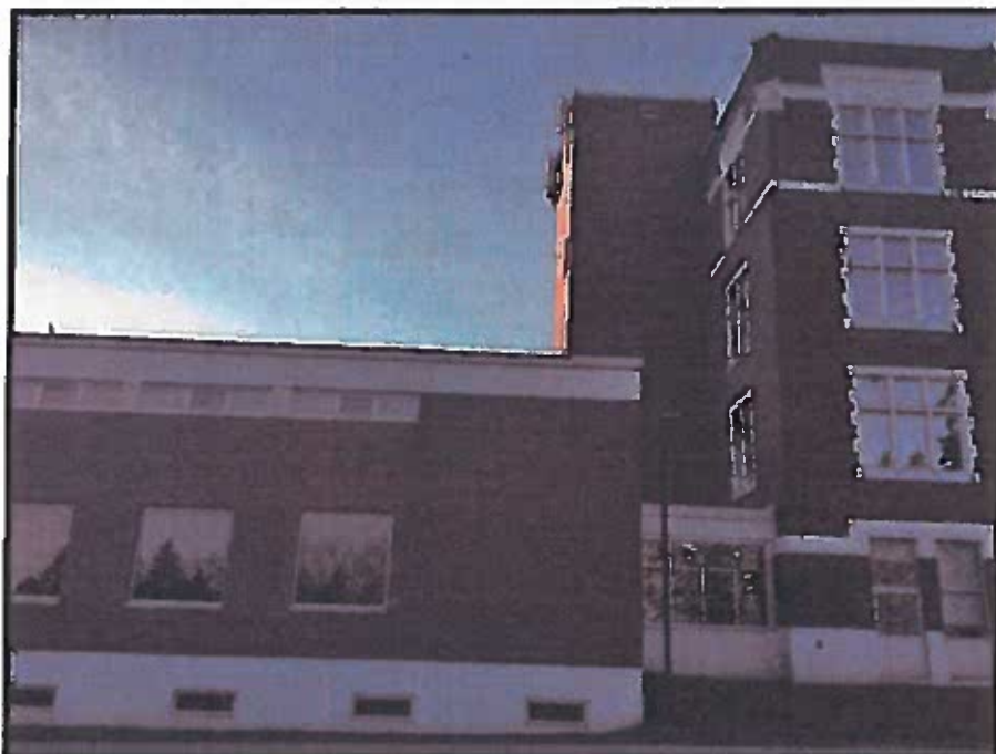
Image 10: Detail of gymnasium addition of former De La Salle College structure (November 27, 2017; View looking West)
