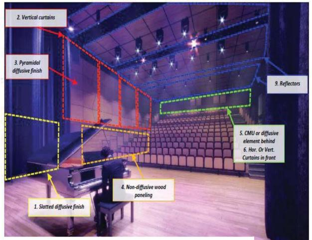
Figure 2. Proposed acoustic finishes within the Multi-Purpose Room
