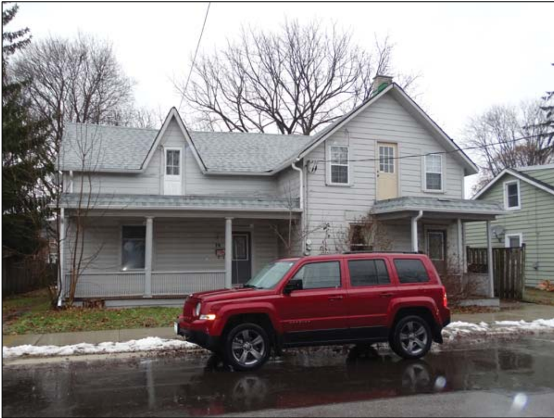
Figure 6: Above: South façade, 2018. The east end of the roof of the west part has been extended to lap into the roof of the east part.
