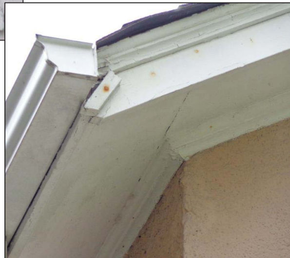
Eave Detail, North-East Corner
