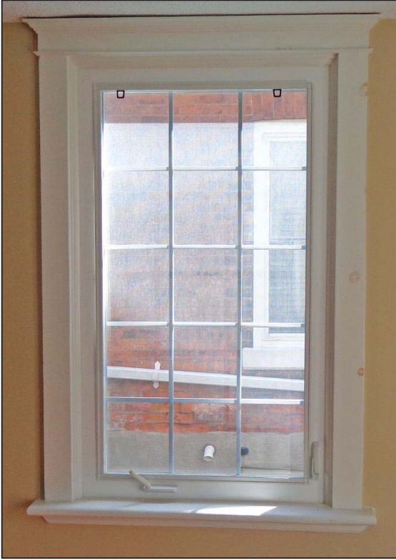
14. Room 2 – Window, East Wall.
