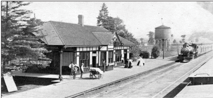
Figure No. 4.2 The Grant Trunk Railway Station in Aurora, circa 1910, [Source, McIntyre, 14].
