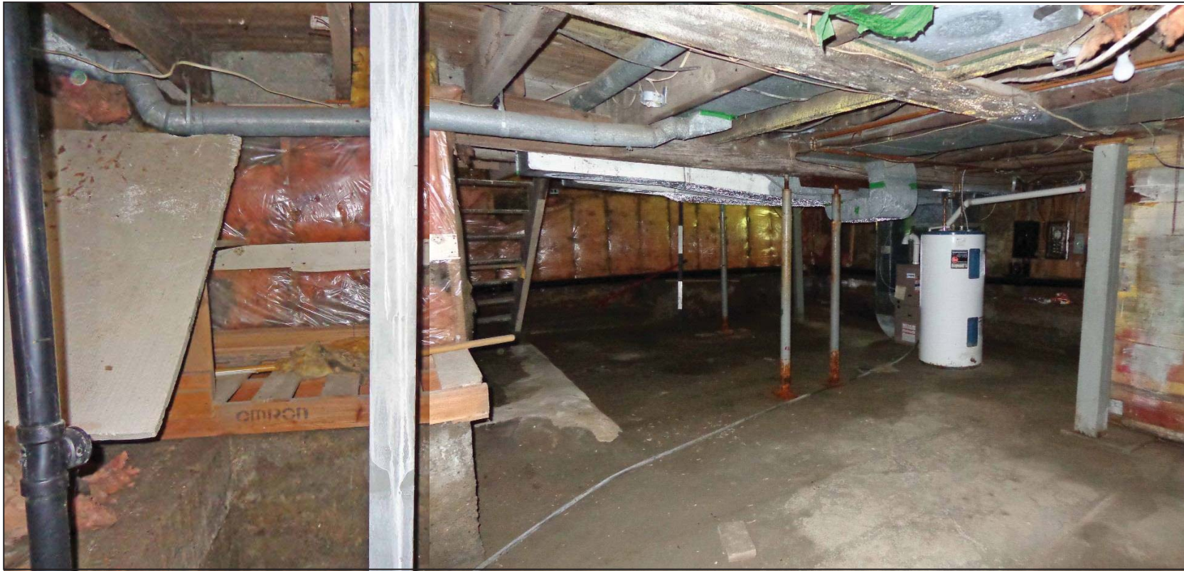
5. View from the southwest corner looking to the north and east walls.
