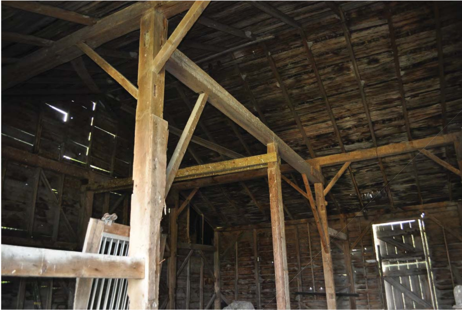
Photo 16: Barn interior (CU 2018).
