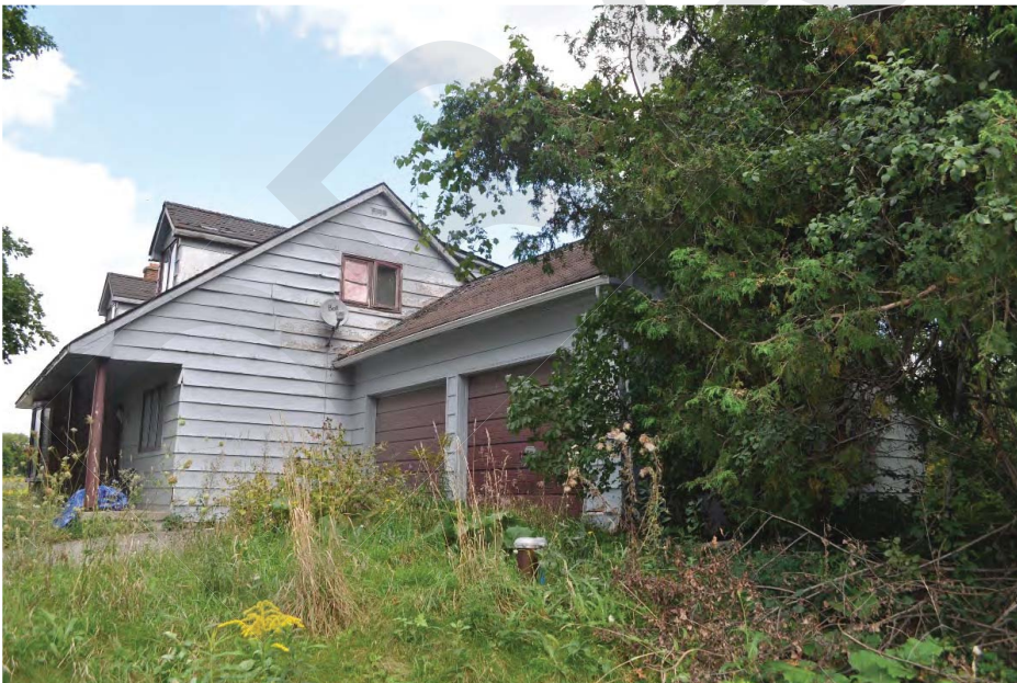
Photo 8: 1625 St. John's Sideroad, south façade (CU 2018).
