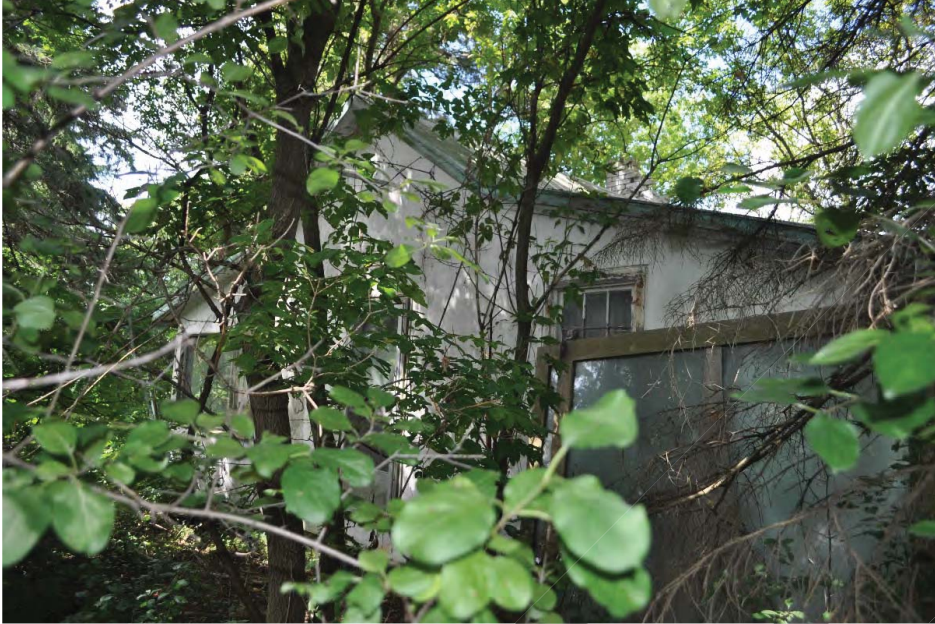
Photo 34: Cottage, south facade (CU 2018).
