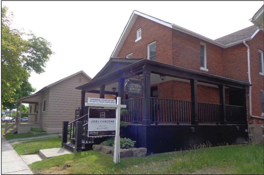
99 and 103 Wellington Street East; buildings immediately east of 97 Wellington Street East.
