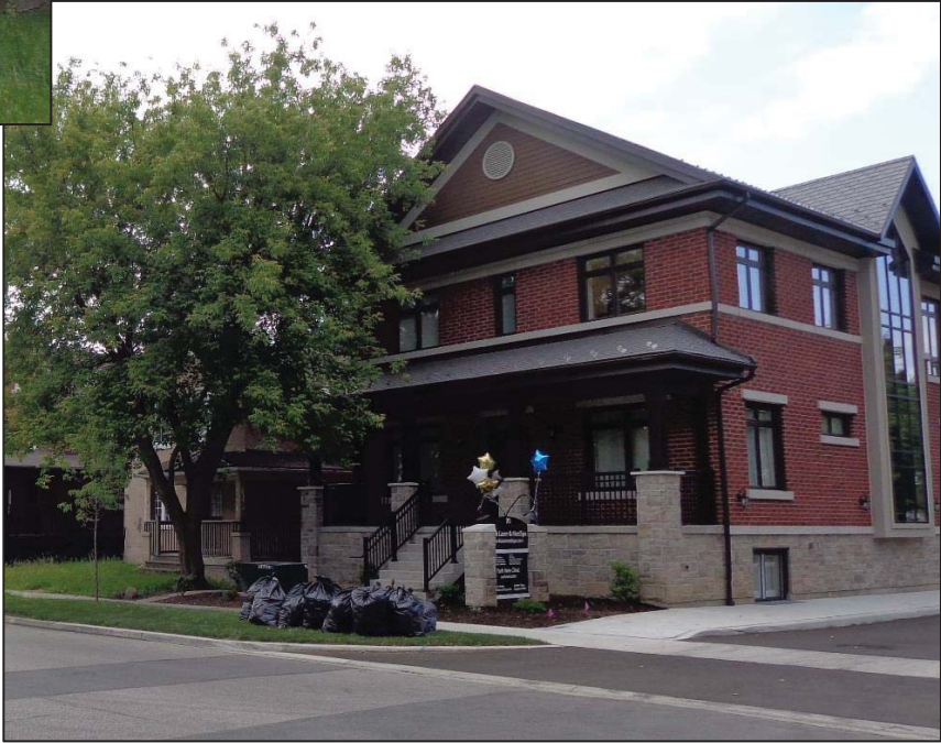
95 Wellington Street East, building immediately west of 97 Wellington Street East.
