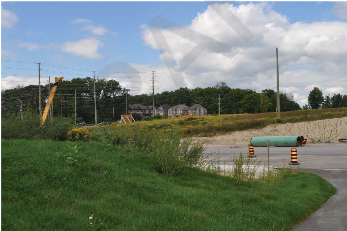
Photo 1: View from 1362 St. John's Sideroad, looking north-northwest towards subdivision west of Leslie Street and north of St. John's Sideroad (CU 2018)
