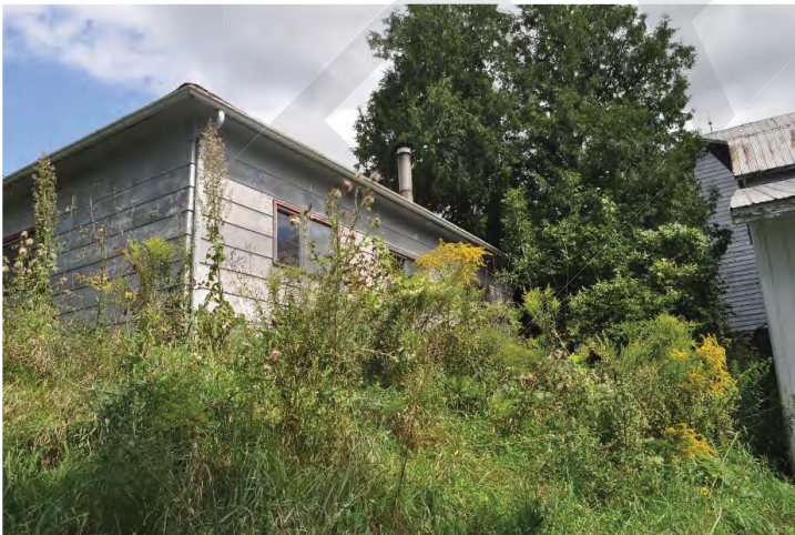
Photo 22: Garage, south elevation (CU 2018).
