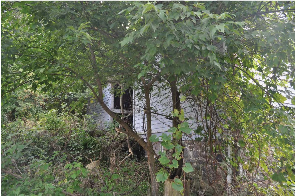
Photo 11: Barn, front (north) facade (CU 2018).
