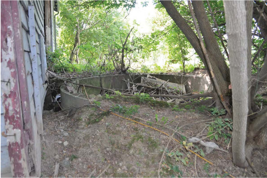
Photo 12: Front (north) of barn, cistern/silo base on right (CU 2018)
