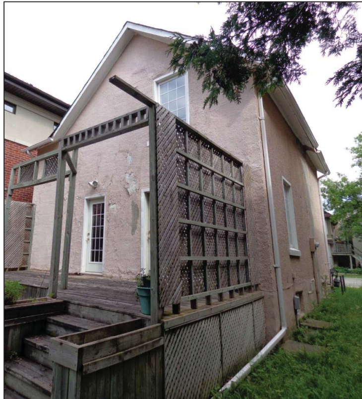
South and East Elevations
