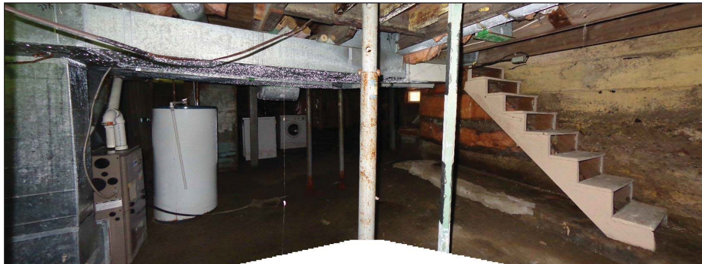
4. South & West Walls.
