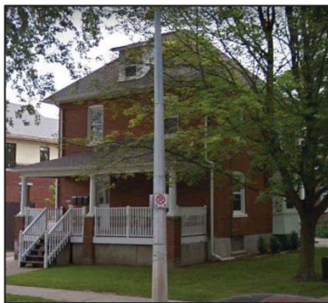
91 Wellington St E North Elevation
