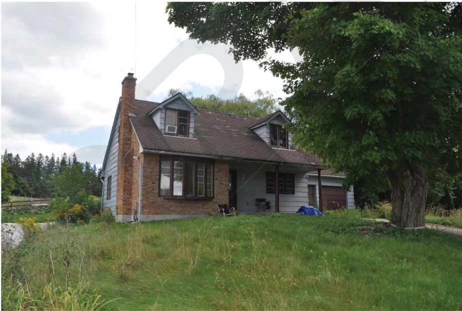
Photo 6: 1625 St. John's Sideroad, west (front) façade (CU 2018).
