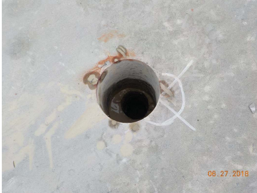
Photo 9 (Looking S): Silty clay found directly below concrete slab in south ramp after CH-6 was removed.
