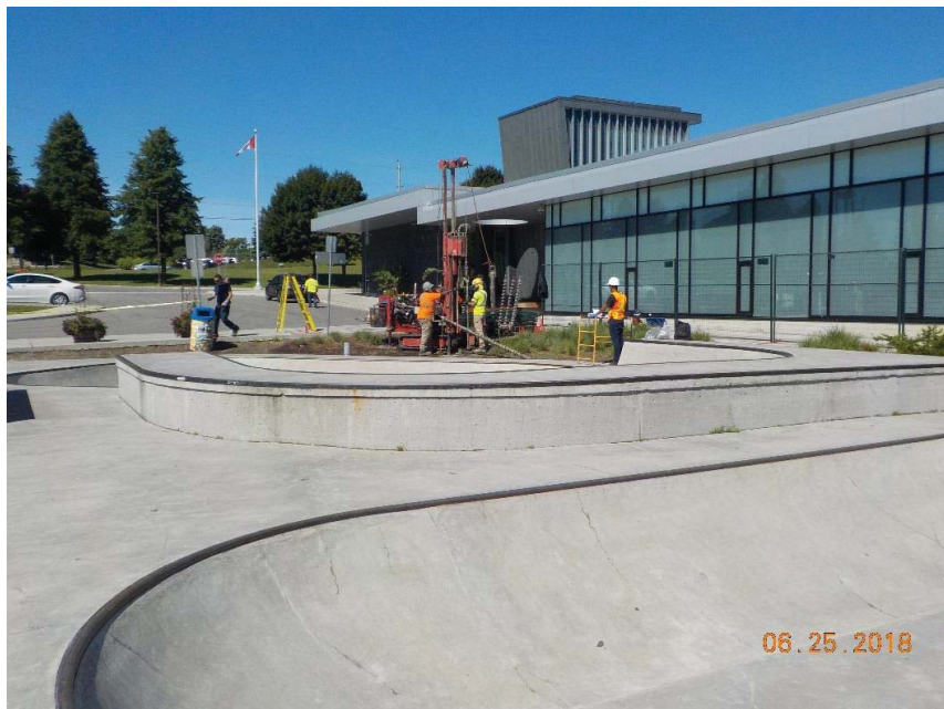
Photo 6 (Looking NW): Geotechnical crew advancing BH-2 in northwest landscaped area.
