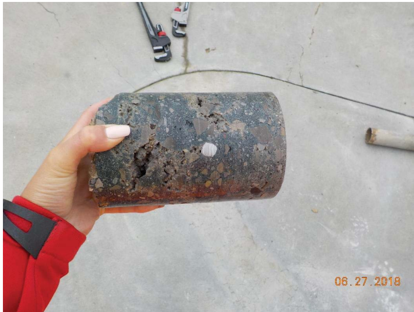
Photo 10 (Looking NW): Rebar sample taken within CH-9.
