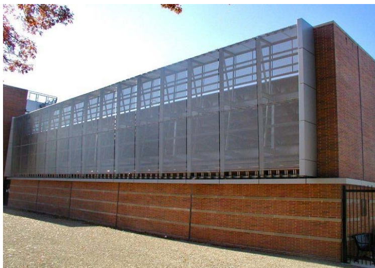
Figure 2 - GKD Mesh Structure Visible
