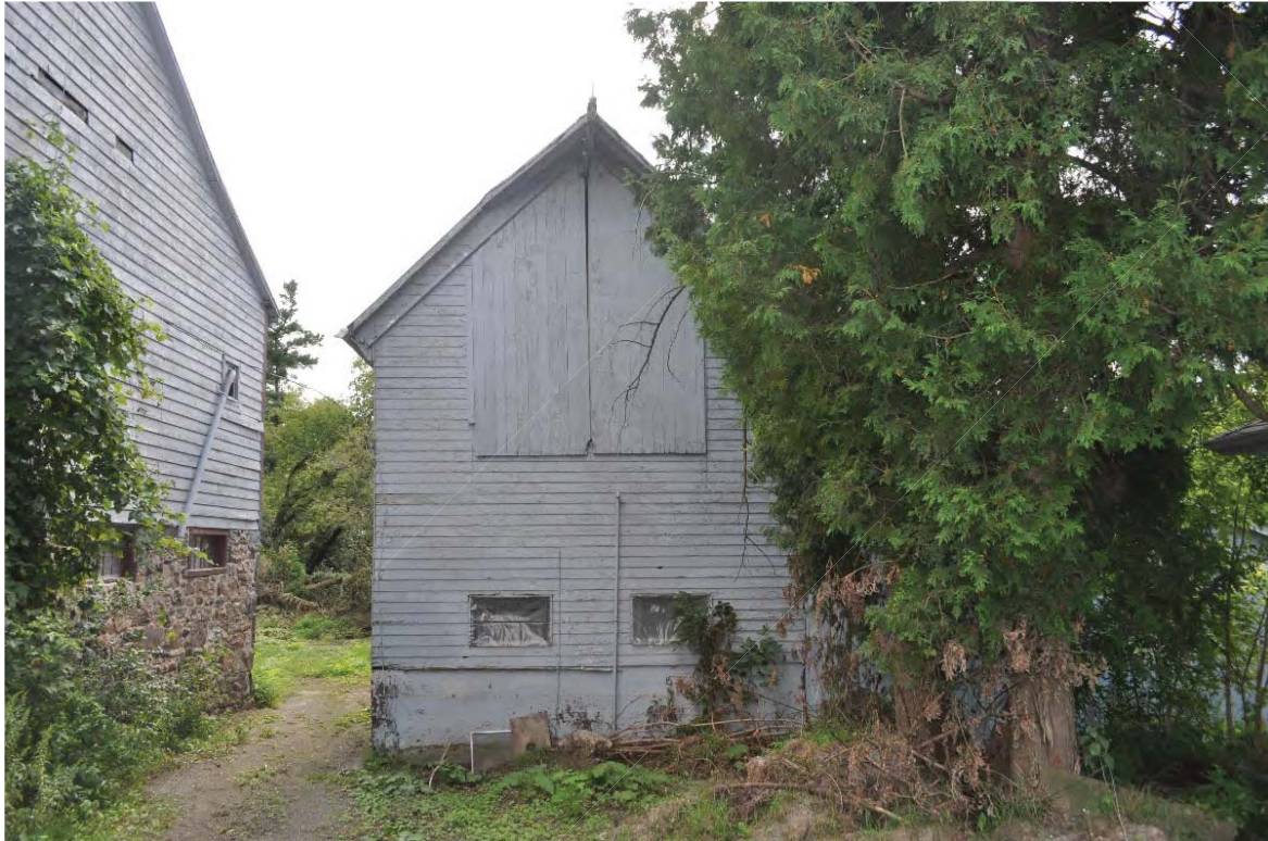
Photo 18: Outbuilding, north facade (CU 2018).
