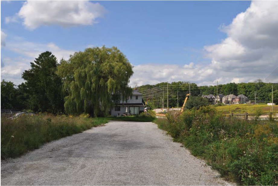
Photo 9: 1625 St. John's Sideroad, east façade from along access road (CU 2018).
