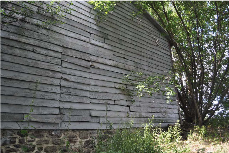
Photo 13: Barn, east facade (CU 2018).
