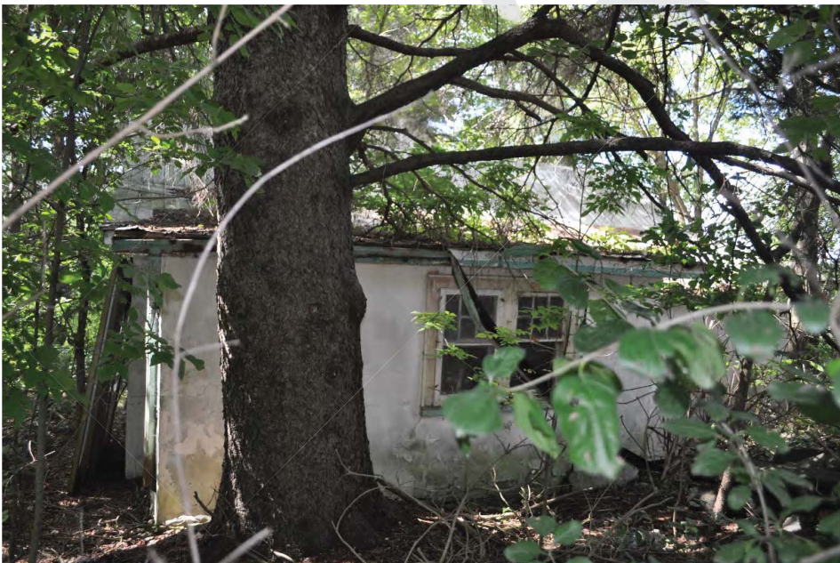
Photo 33: Cottage, east facade (CU 2018).
