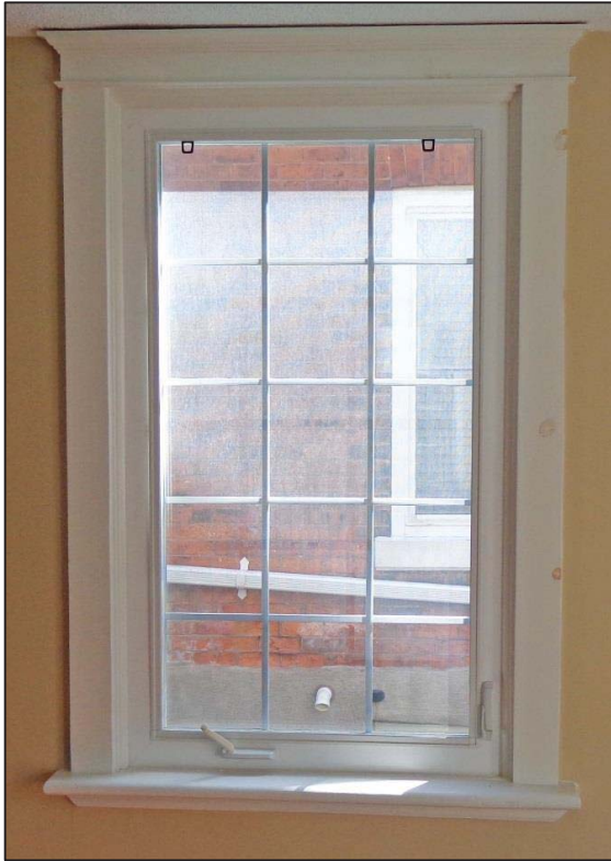
14. Room 2 – Window, East Wall.
