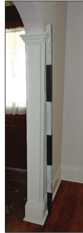
7. Room 1 – Pilaster on opening to Hall.
