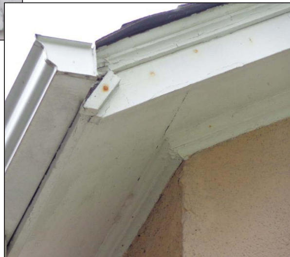
Eave Detail, North-East Corner
