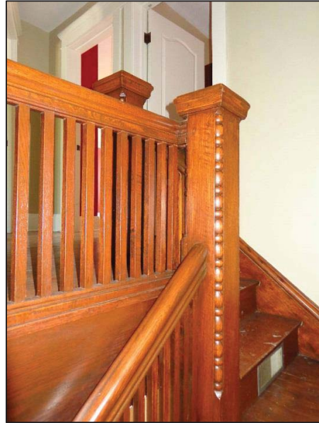
Figure 5.2 House, 97 Wellington Street East, staircase
