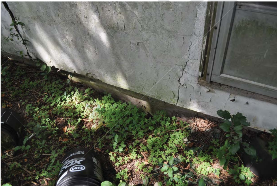
Photo 37: Cottage, detail of cladding (CU 2018).
