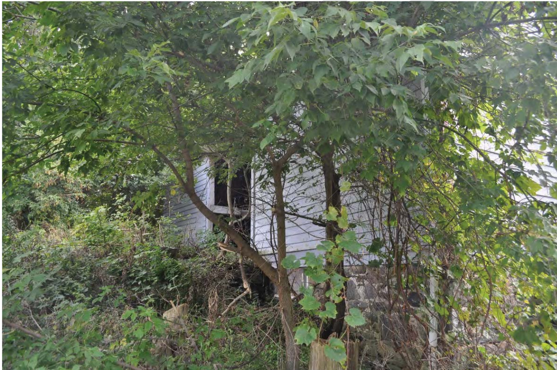
Photo 11: Barn, front (north) facade (CU 2018).
