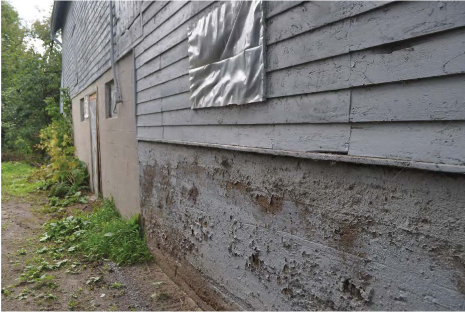
Photo 19: Outbuilding, east elevation foundations (CU 2018).
