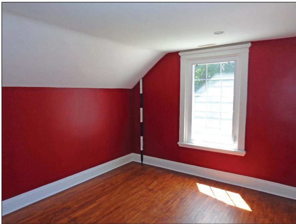
9. Room 2 – East and South Walls.
