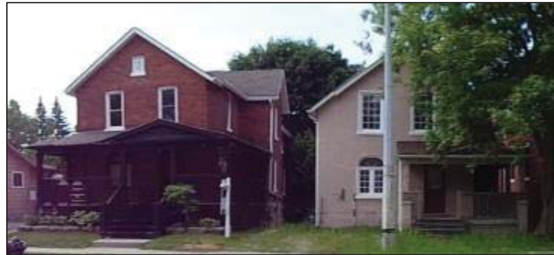
Figure 6.1 99 (left) & 97 (right) Wellington St E, 2018.
