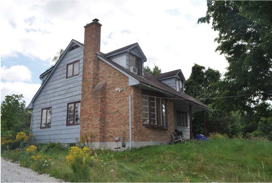
Photo 5: 1625 St. John's Sideroad, north façade (CU 2018).
