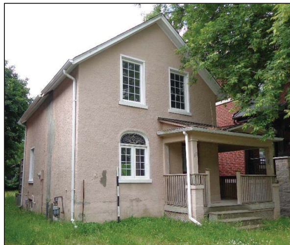
Figure 5.1 House at 97 Wellington Street East, East and North Elevations, 2018
