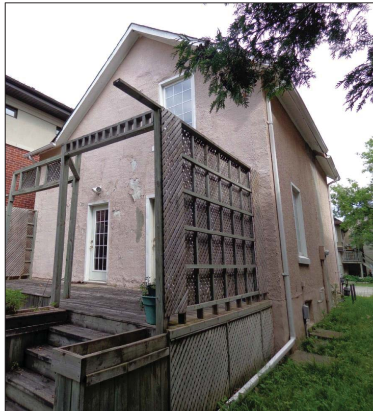
South and East Elevations
