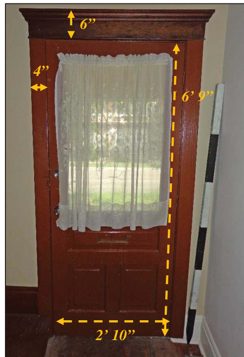
1. Hall – Front Door.
