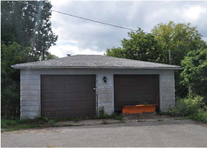
Photo 21: Garage, north elevation (CU 2018).
