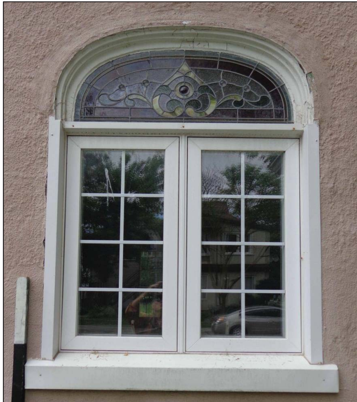
Ground Floor Window, North Elevation
