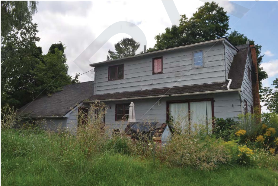
Photo 10: View of 1625 St. John's Sideroad, rear (east) façade (CU 2018).
