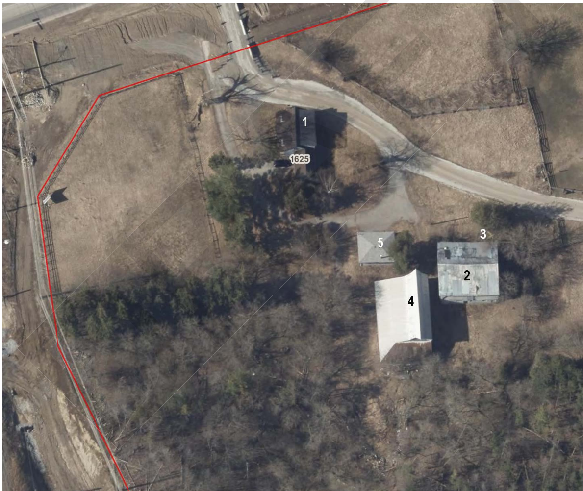
Figure 8: 1625 St. John's Sideroad, current conditions (base map source: YorkMaps, 2018)
