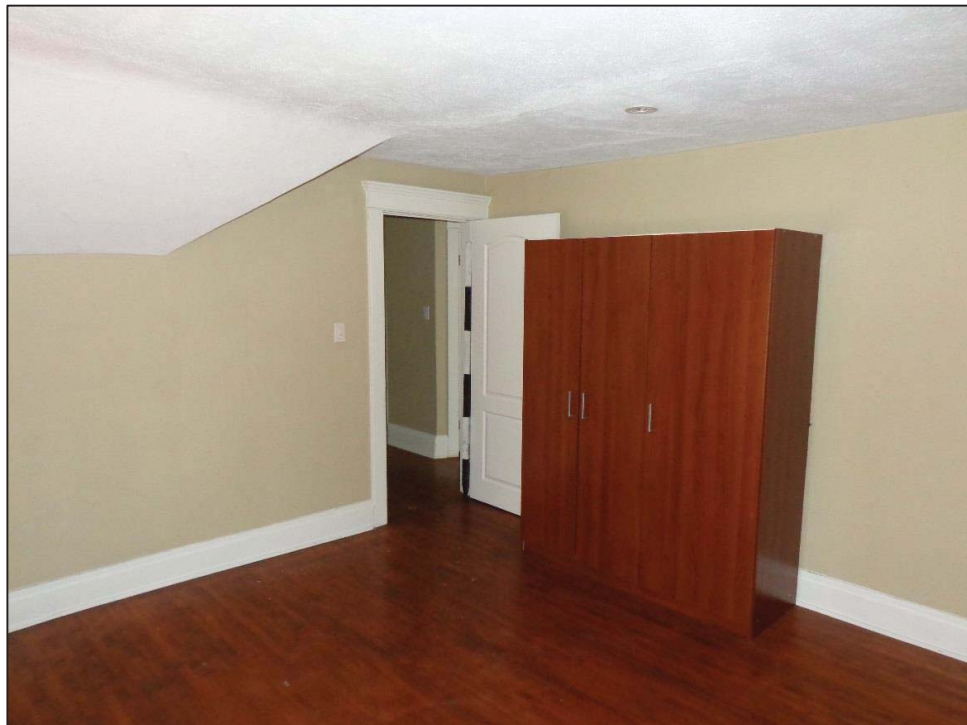
4. Room 1 – North and East Walls.
