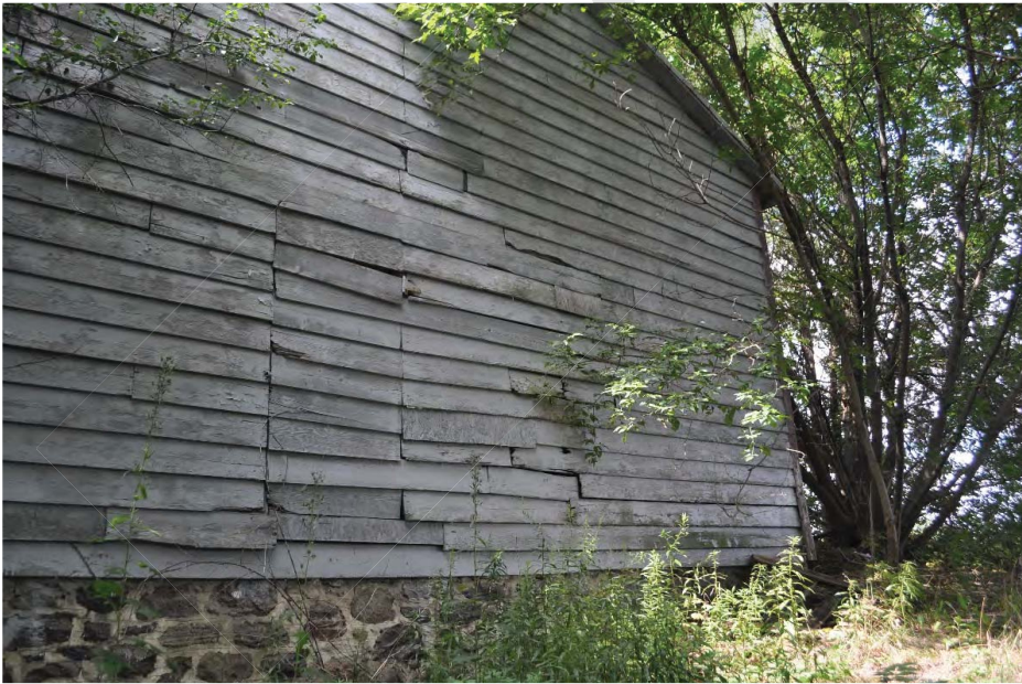
Photo 13: Barn, east facade (CU 2018).
