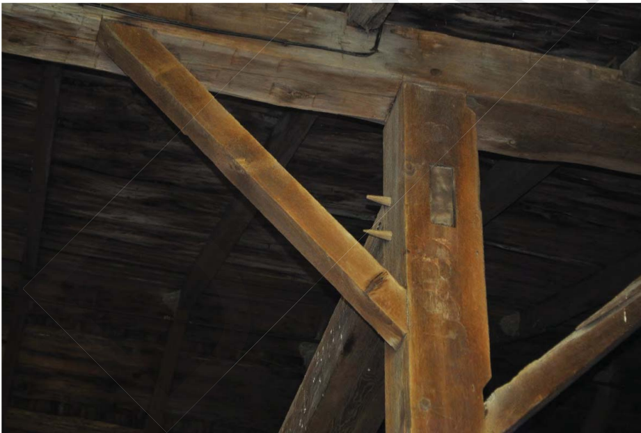
Photo 17: Detail, barn interior (CU 2015).
