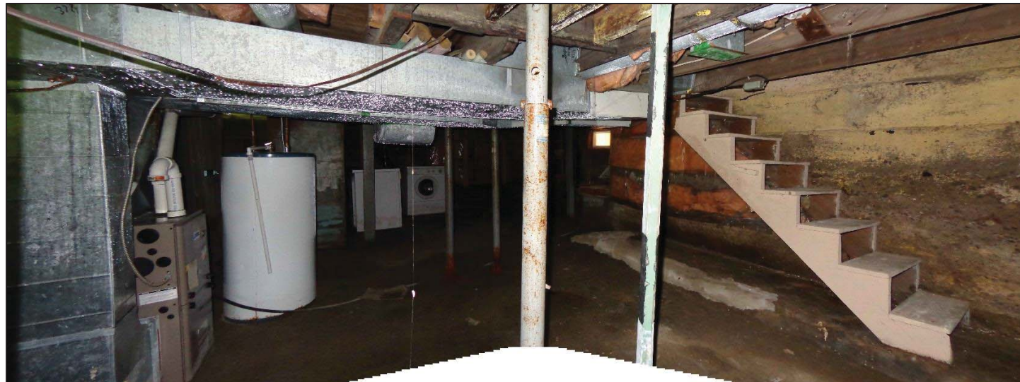
4. South & West Walls.
