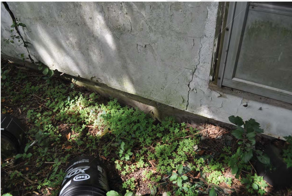
Photo 37: Cottage, detail of cladding (CU 2018).
