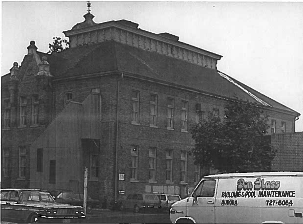
Southwest view of the school showing fire escape at east elevation, date unknown (Aurora Archives).
