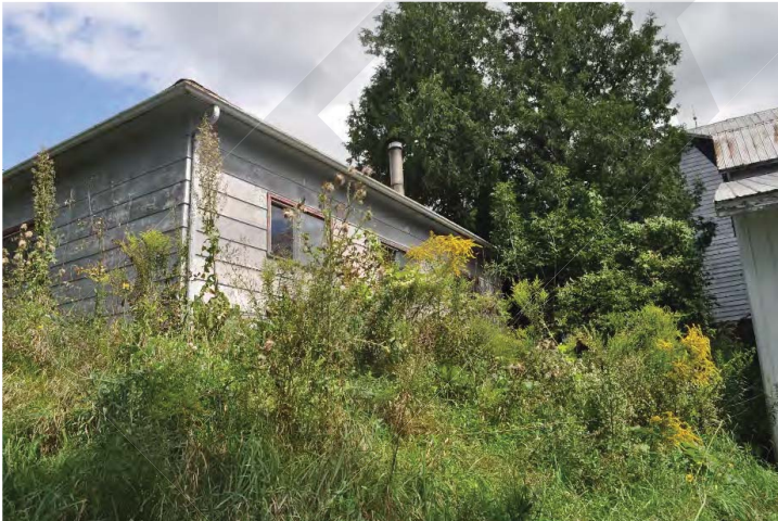
Photo 22: Garage, south elevation (CU 2018).
