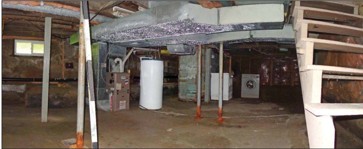
3. East & South Walls.
