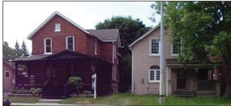
Figure 6.1 99 (left) & 97 (right) Wellington St E, 2018.
