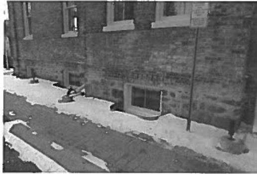
Foundation and basement windows at east elevation (ERA, 2019).
