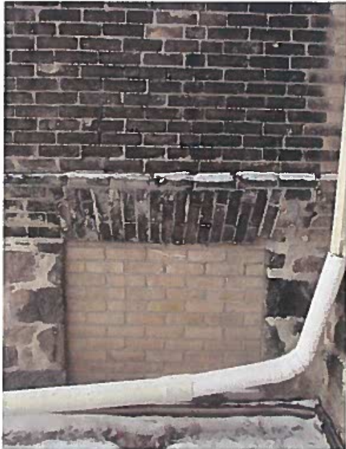
Bricked in window at the south elevation (ERA, 2019).
