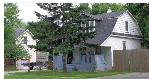
Figure 6.2 95 - 103 Wellington St E (above), 95 Wellington St E (right), 2013.
