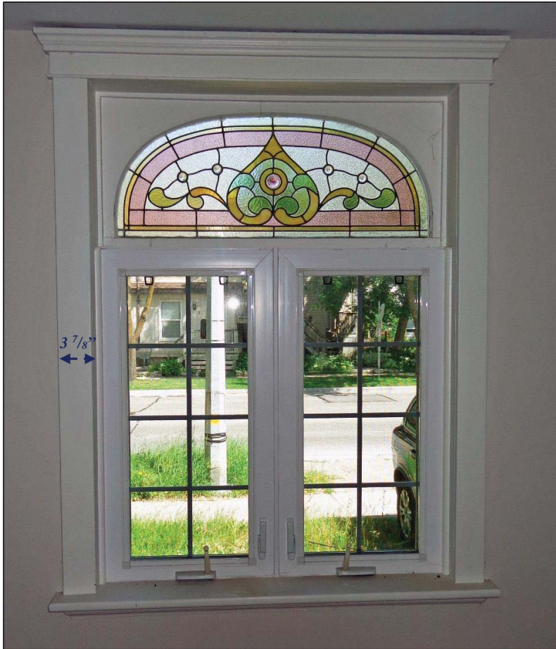
10. Room 1 – Window on North Wall.
