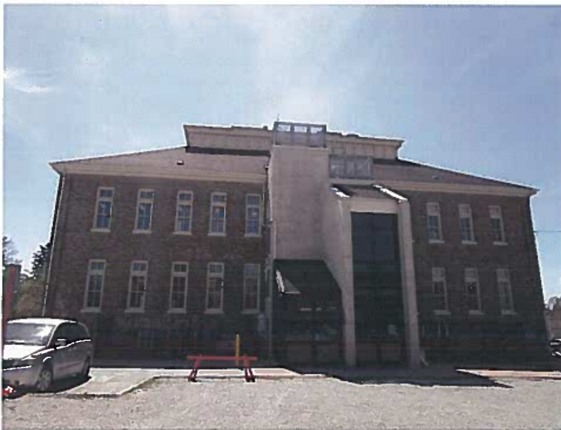
North elevation of 22 Church Street (ERA, 2018).
