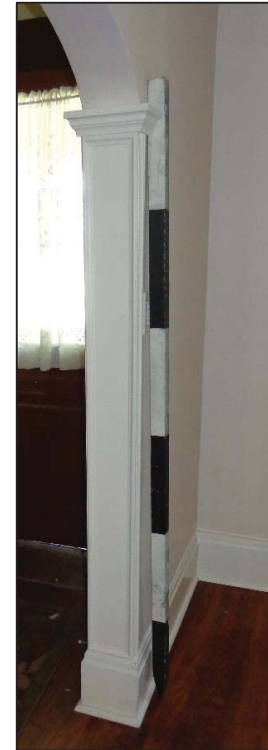
7. Room 1 – Pilaster on opening to Hall.
