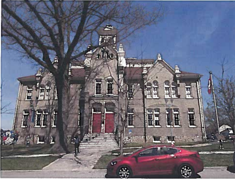
South elevation of 22 Church Street (ERA, 2018).
