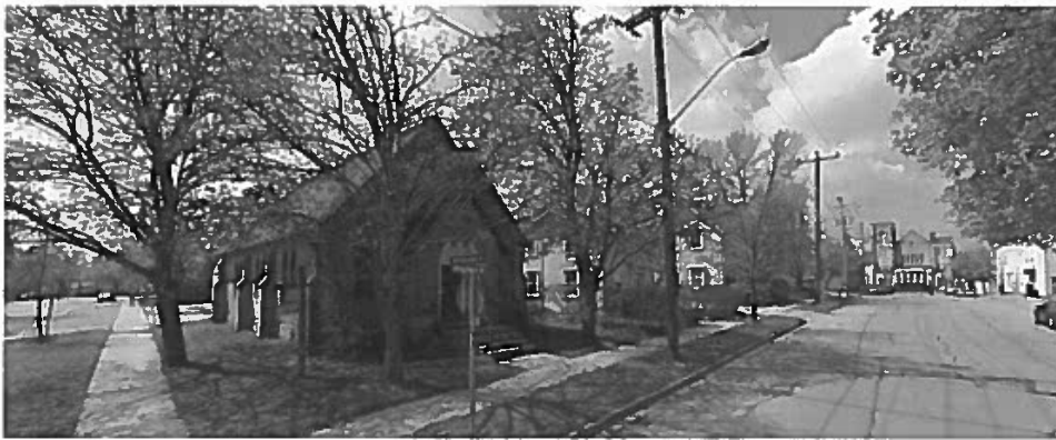
View looking west on Mosley Street showing properties at 11-27 Mosley Street (Google Images, 2019).
