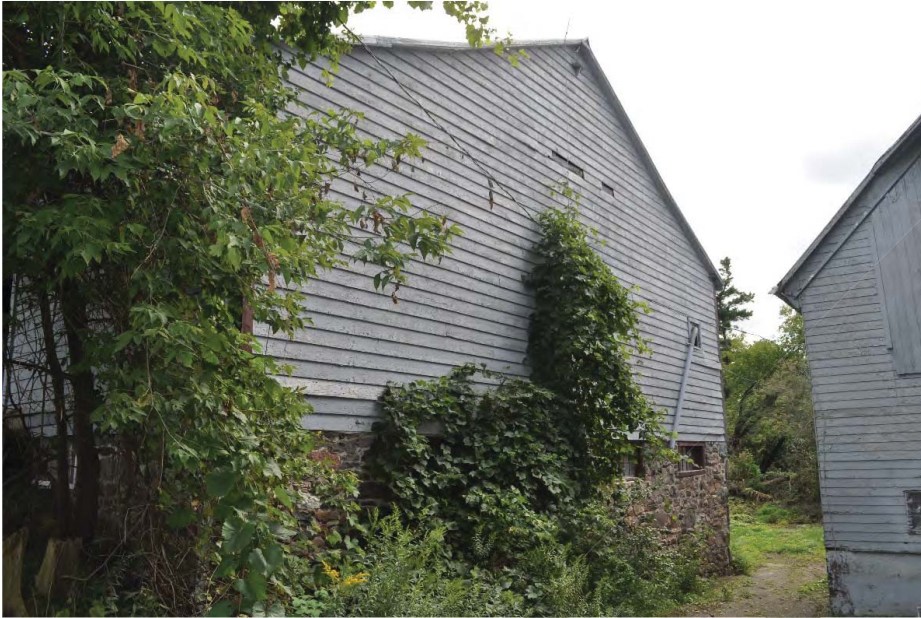
Photo 14: Barn, west facade (CU 2018).
