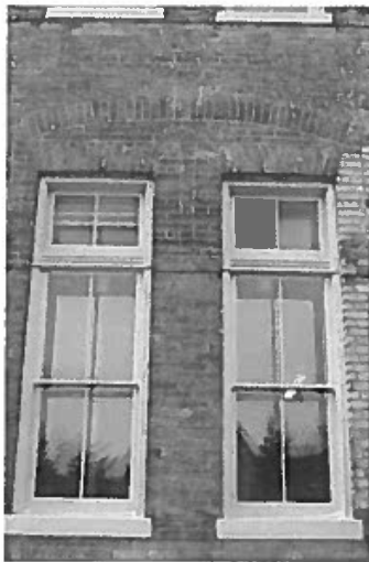
Windows at east elevation (ERA, 2019).
