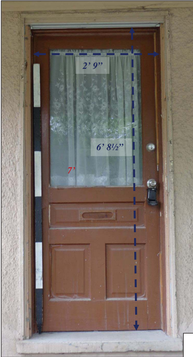
Front Door, North Elevation
