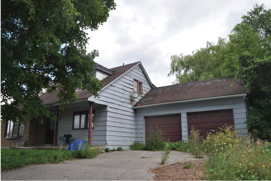
Photo 7: 1625 St. John's Sideroad, west (front) façade, showing attached two-car garage (CU 2018).
