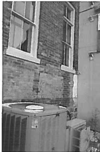
Detail of brick at north elevation (ERA, 2019).
