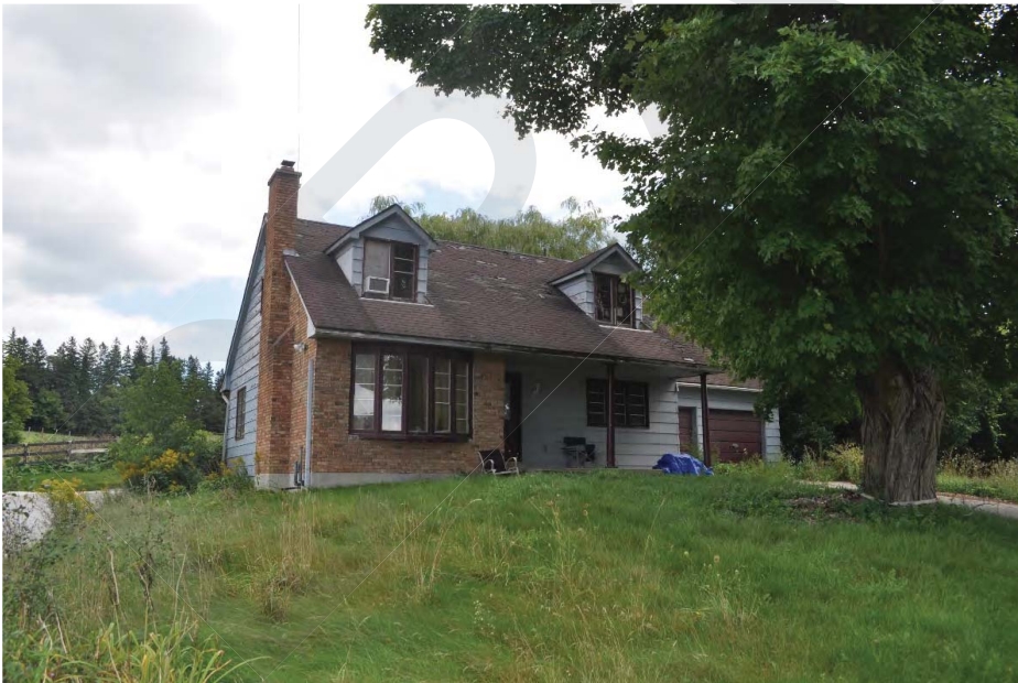
Photo 6: 1625 St. John's Sideroad, west (front) façade (CU 2018).
