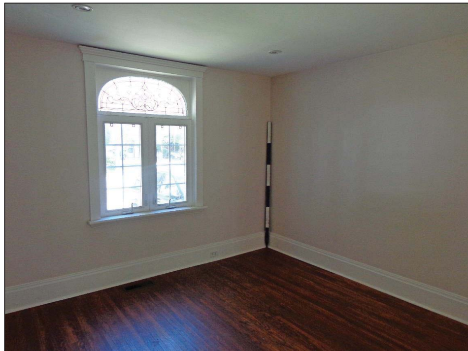
9. Room 1 – North and East Walls.
