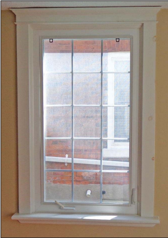
14. Room 2 – Window, East Wall.
