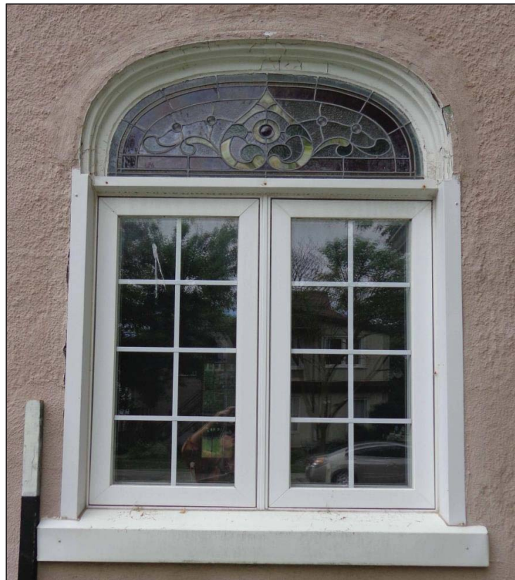
Ground Floor Window, North Elevation
