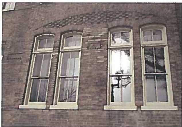
Windows at the south elevation (ERA, 2019).
