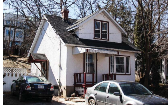
Figure 19 - View to north corner (Photo: RHC 2019)
