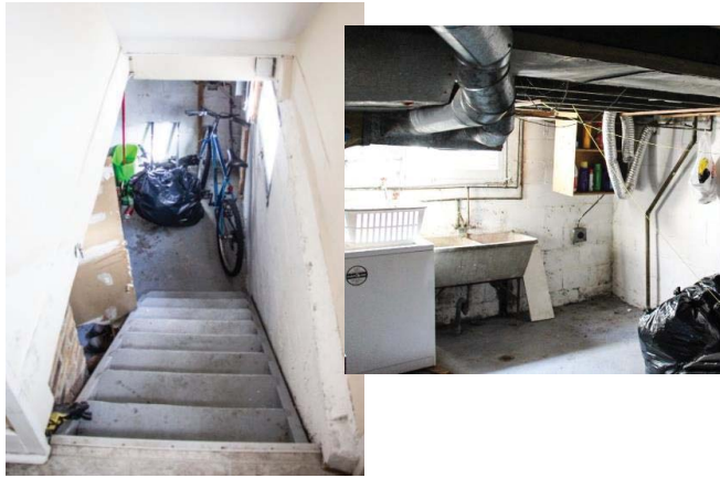
Figure 32 - Basement stair; concrete laundry sink under basement window. (Photo: RHC 2019)
