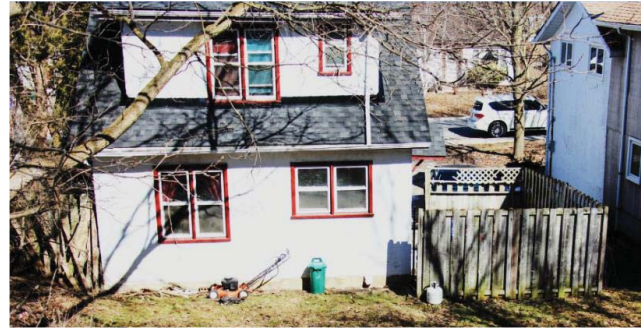
Figure 23 - View from slope at rear. (Photo: RHC 2019)
