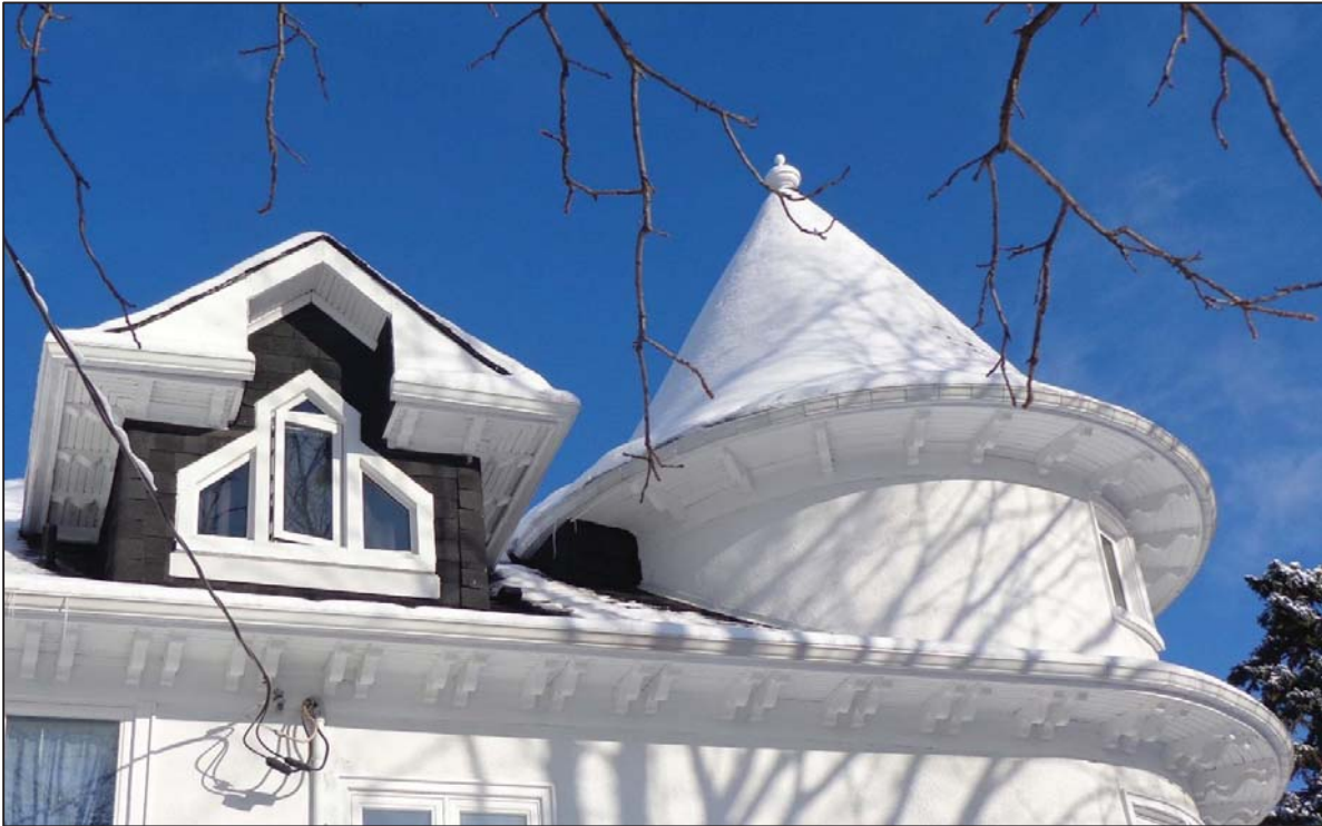
Dormer and Corner Tower, South Elevation.
