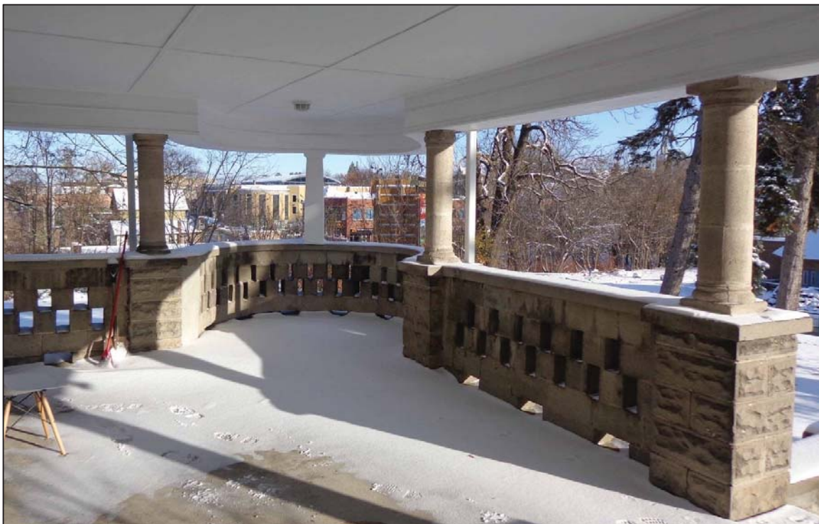
Interior Veranda Detail, North & East Elevations.
