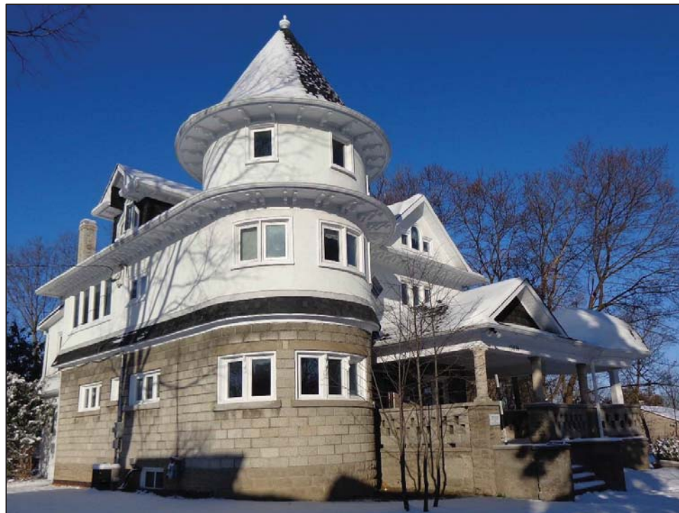
South and East Elevations
