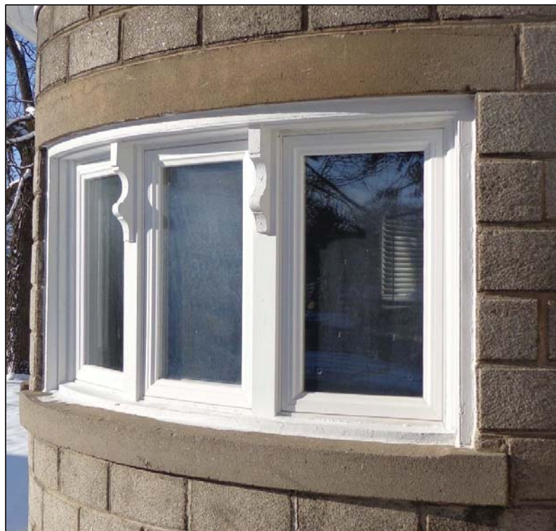
Ground Floor Tower Window Detail, East Elevation.
