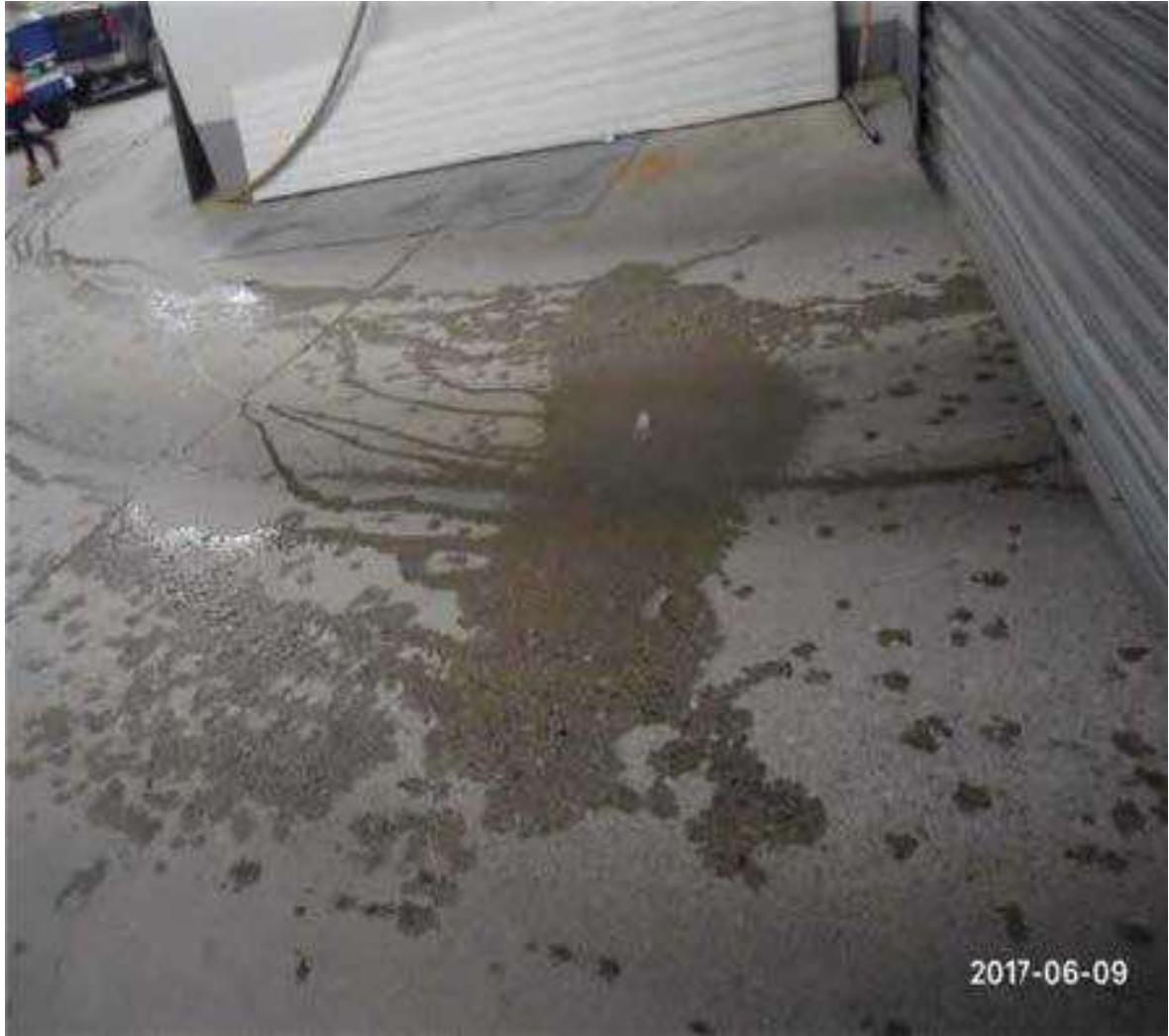
unfinished concrete floor.jpg
