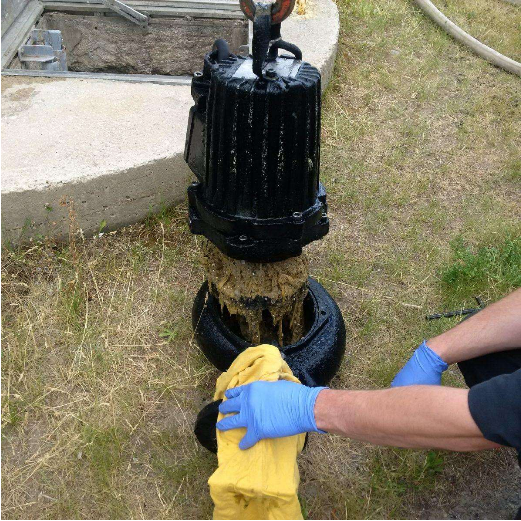
C:\Users\Jim Tree\Desktop\Ballymore pump cleaning June 27th 2016 (5) (002).jpg
