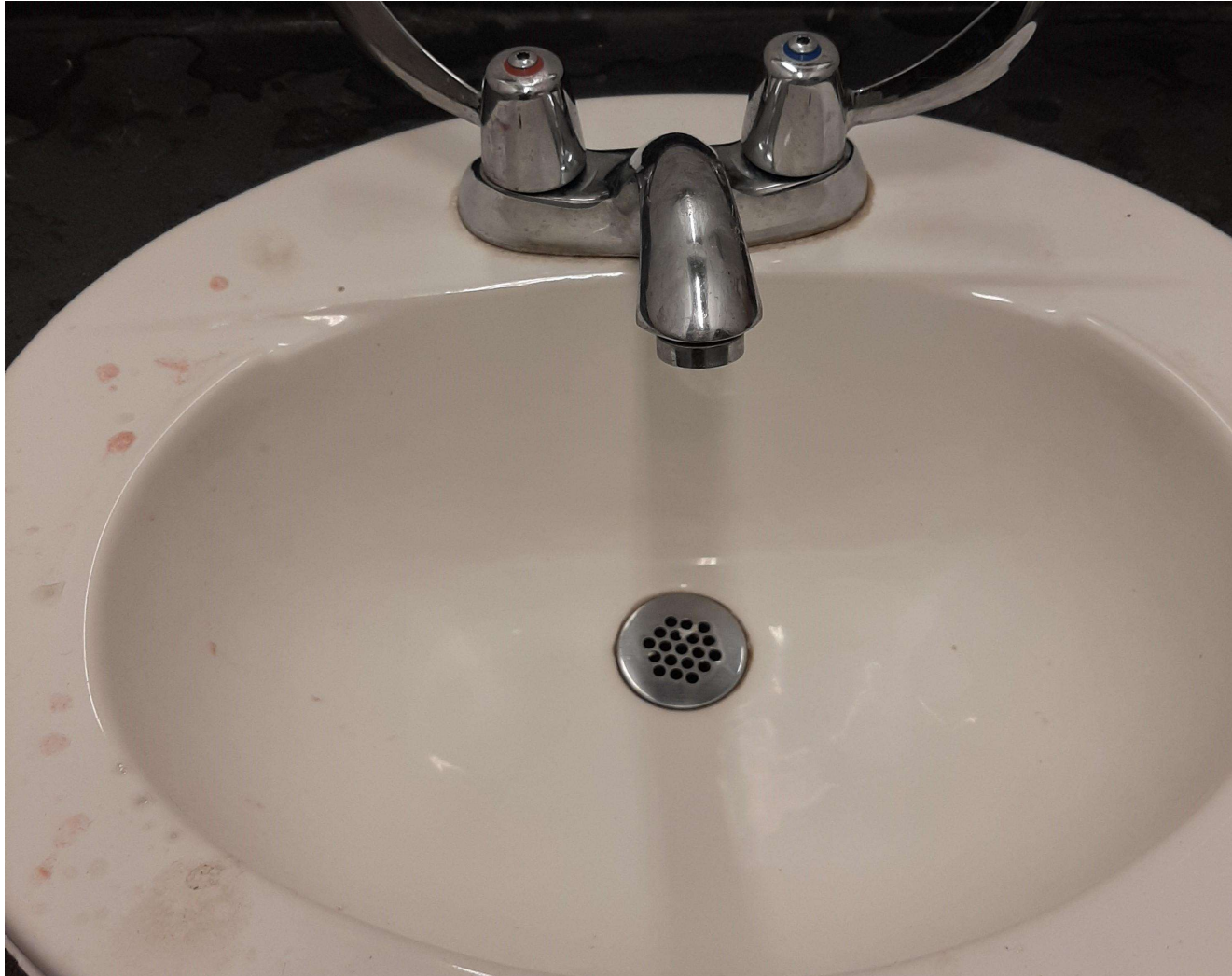
C:\Users\Doug Bertrand\Pictures\Budget Sheet Pictures\SARC - Plumbing Fixtures (3).jpg
